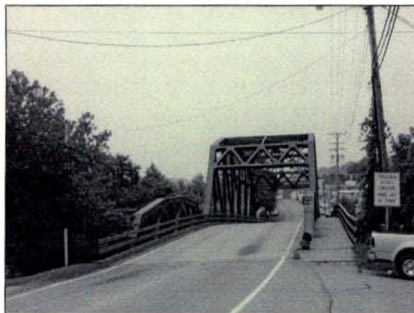
Photograph of bridge from northern approach heading into Gassaway.
