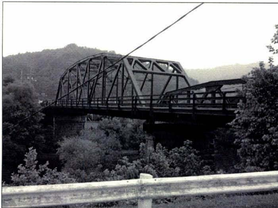
Photograph of bridge showing supports, facing northeast.
