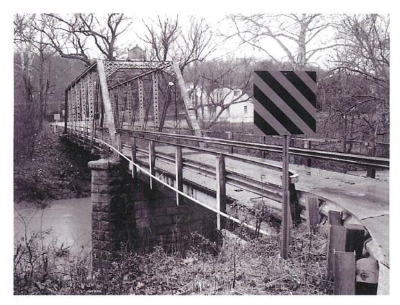
The existing bridge was built in 1888, consists of two pins connected single span, with an overall length of 156 feet. The bridge was reinforced in 1954 and renovated in 1980 by the Department of Highways. The last renovation allows for the posted load limit of 15 tons.
