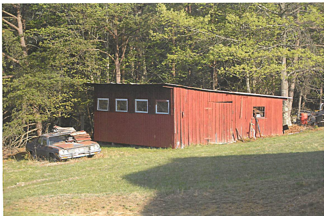
Clark/Racey Farmstead, Poultry House, Facing N
