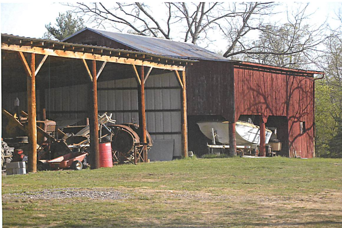
Clark/Racey Farmstead, Machine Shed and English Barn, Facing NE
