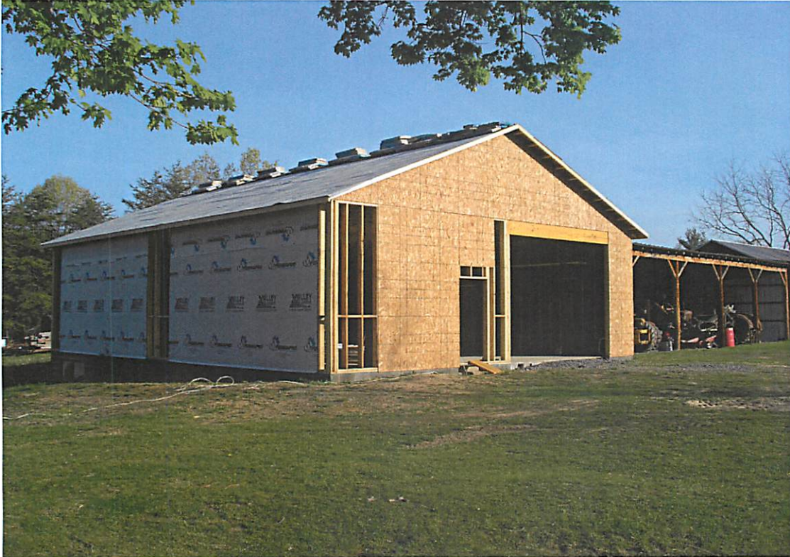
Clark/Racey Farmstead, Garage Construction, Facing NE
