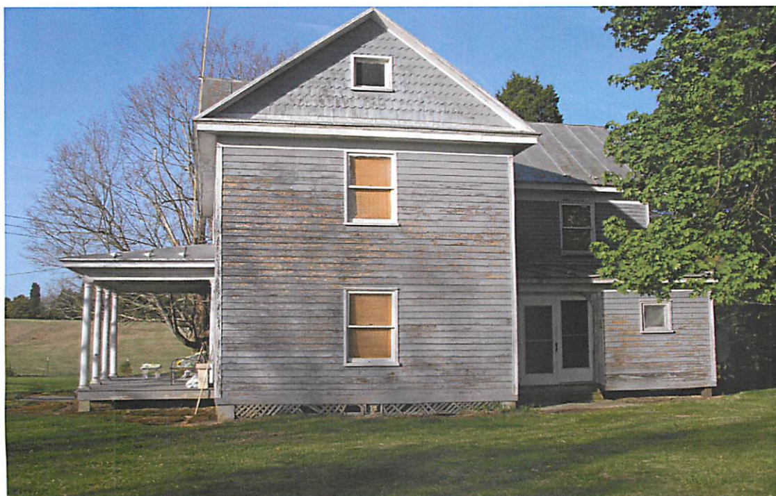
Clark/Racey Farmstead, Main Dwelling, East Elevation, Facing W
