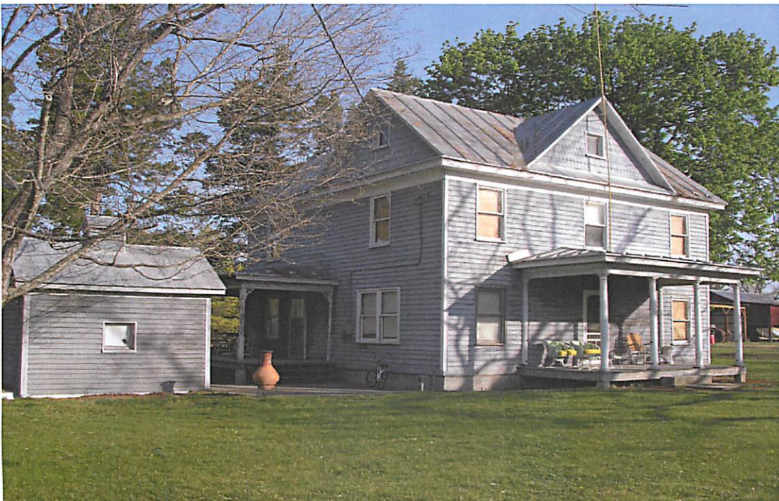
Clark/Racey Farmstead, Main Dwelling, Facing NE
