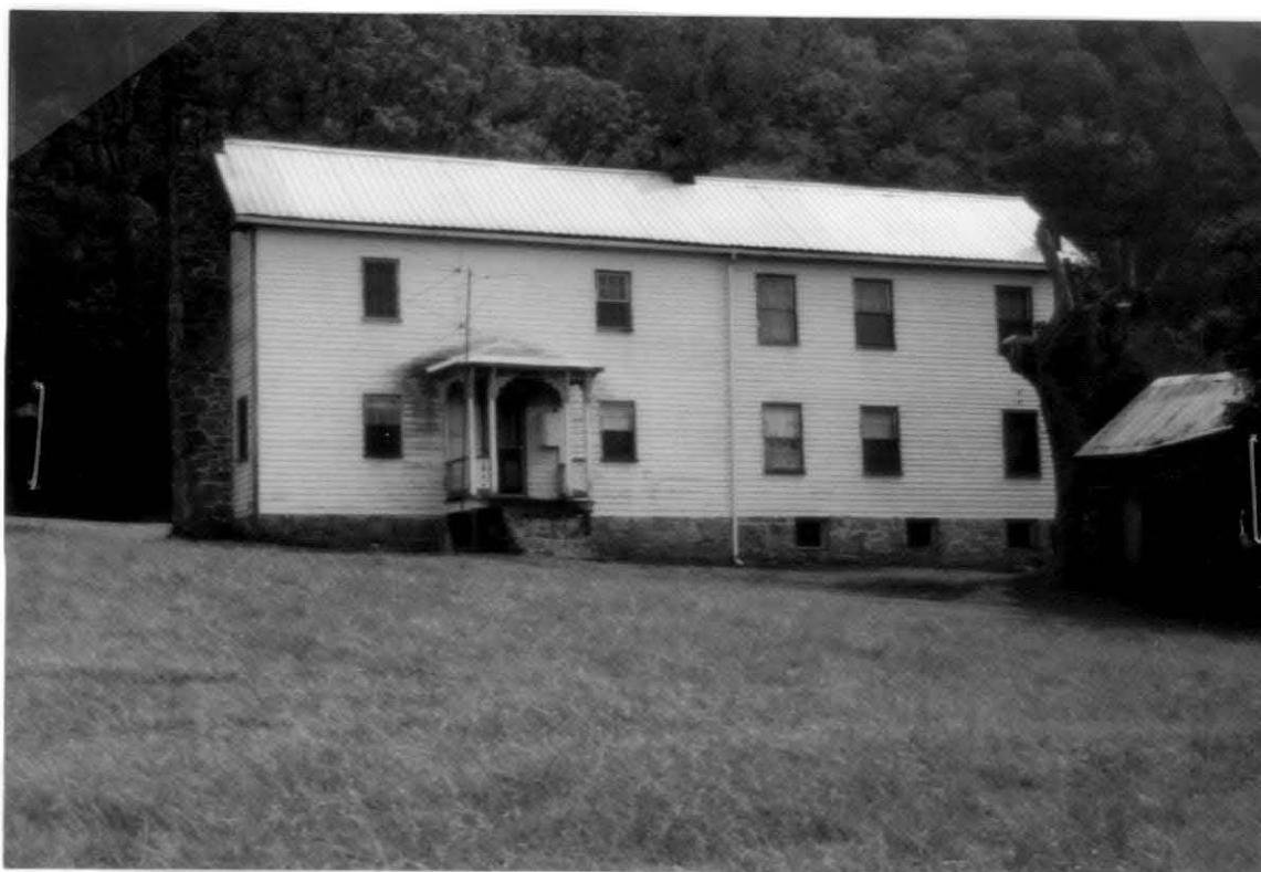
Photo # 3 Second section on right of "enclosed log cabin".
