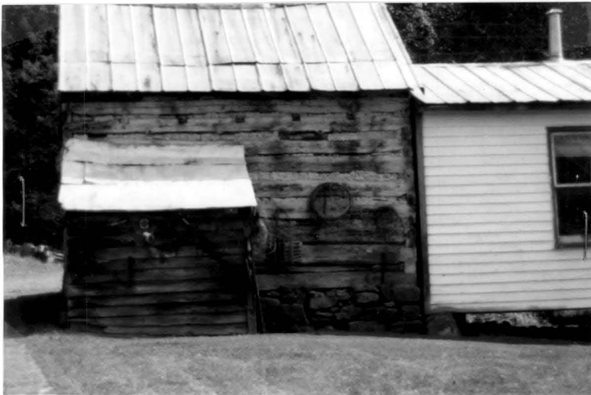
Photo #10 Southern profile of outbuildings #9-10.
