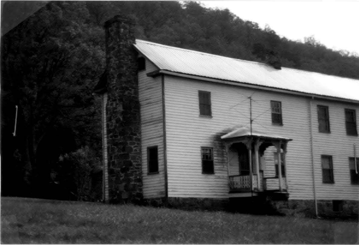
Photo # 1 Parker House original section looking northwest from present Rt. 50.
