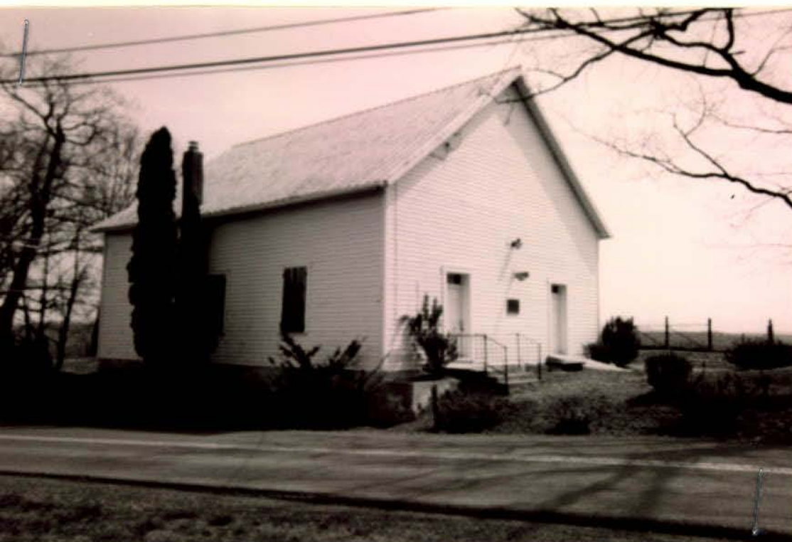
Mount Bethel Church front entrance (South) and West side.
