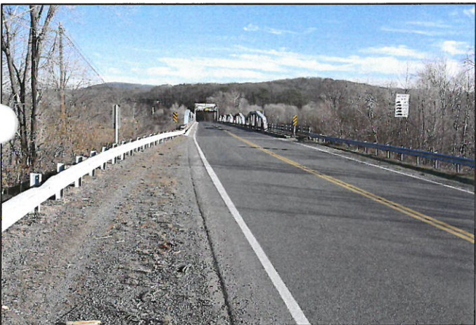
Immediate Approach to Romney Bridge from West, Facing East
