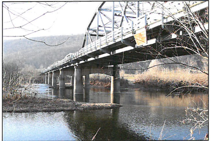
View of Upstream Side of Bridge and Piers, Facing West
