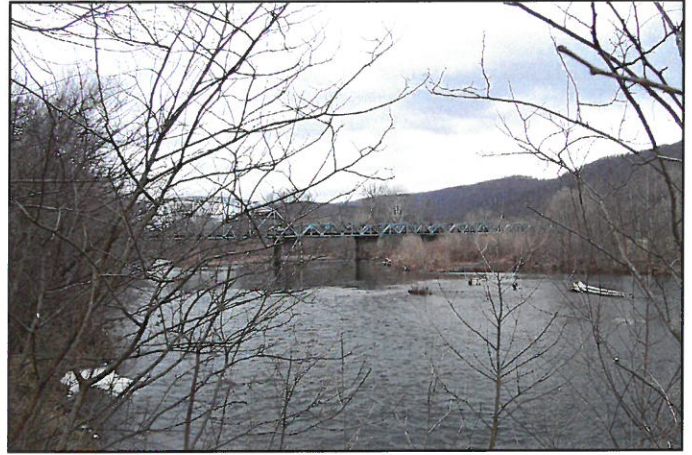
Spans and South Branch of Potomac River, Facing South
