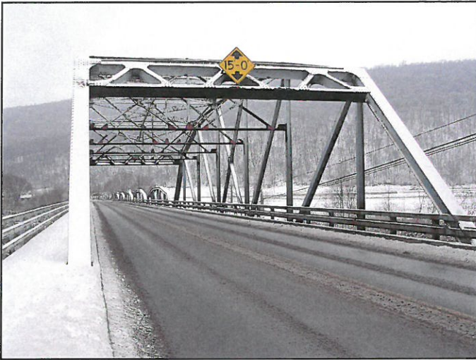
Detail View of Camel-Back Truss, Facing West
