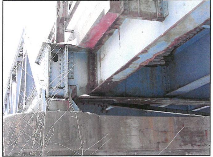
Detail View-Rocker Bearing Connection, Facing Southeast
