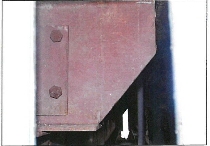
Detail View of Replacement Support Members
