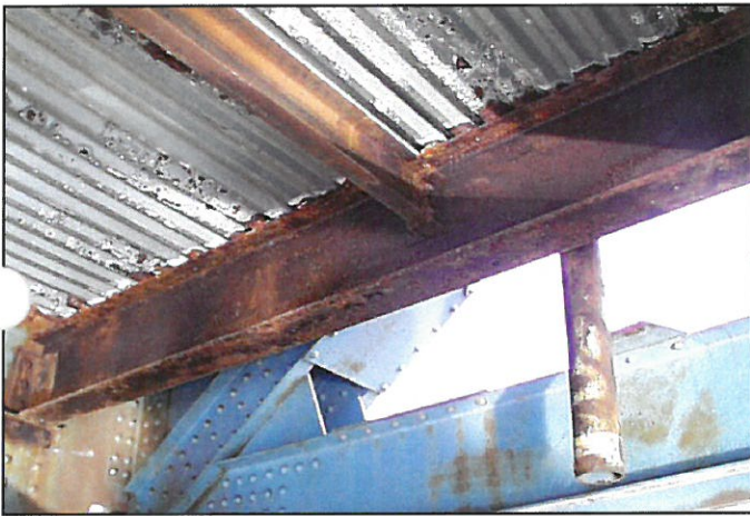
Detail View of Deck Repairs from Underside
