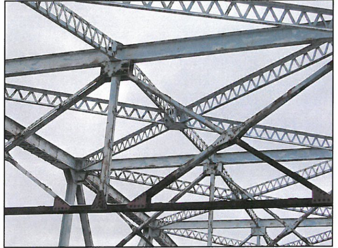
Detail View of Top Chord Bracing, Facing Northeast
