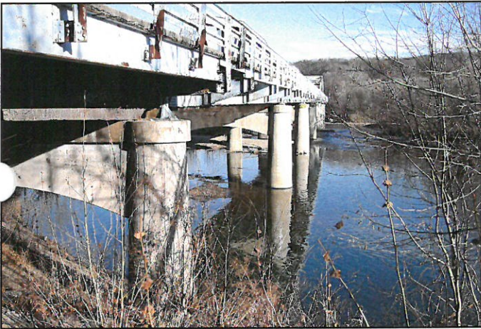
View of Bridge Piers and Walkway, Facing East
