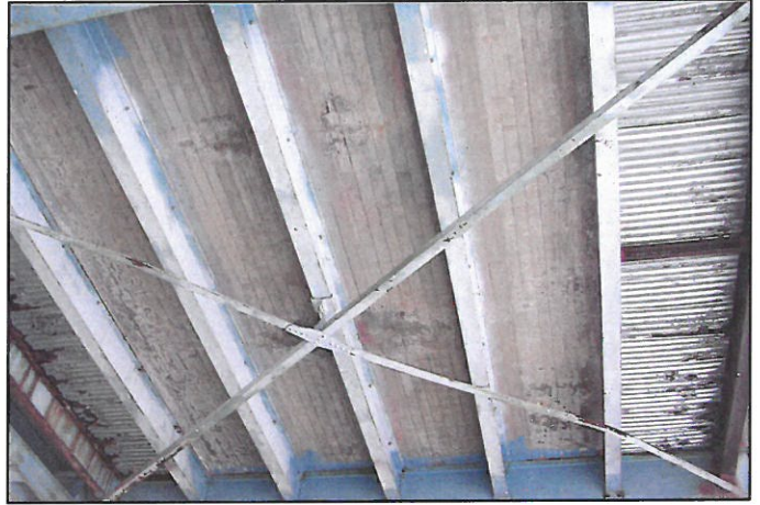
Detail View of Repaired Span
