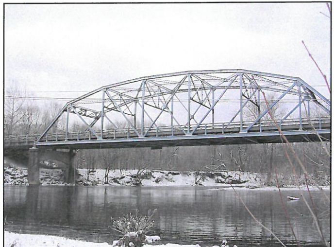
View of Main Span from Downstream, Facing South
