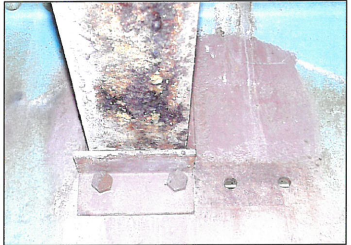
Detail View of Repaired Connections
