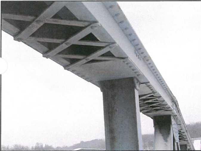
Detail View of Lattice Bracing, Facing East
