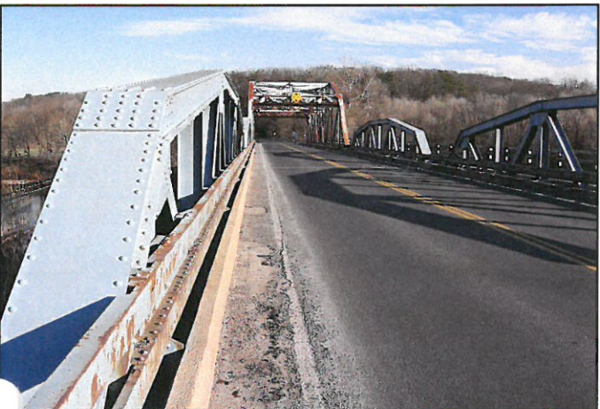
View of Pony Trusses and Camel-Back Truss, Facing East
