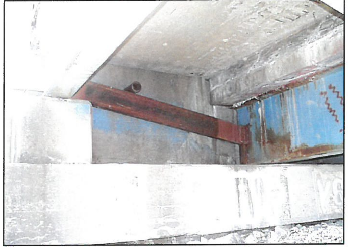
Detail View of Supplemental Bracing Replacement
