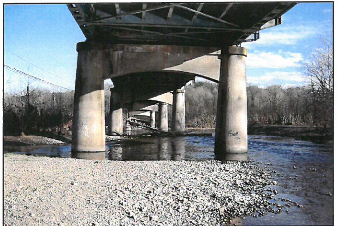
Detail View of Piers under Bridge, Facing East
