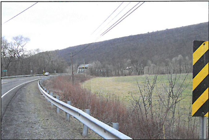
Romney Bridge Showing Approach, Facing West-Southwest
