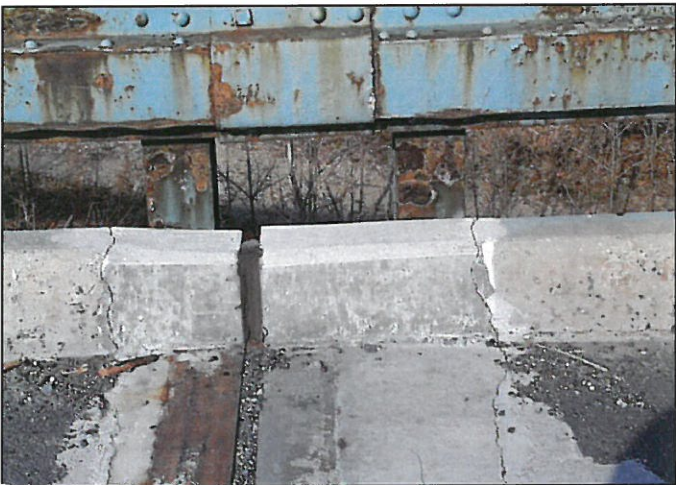
Detail View of Repaired Expansion Joints
