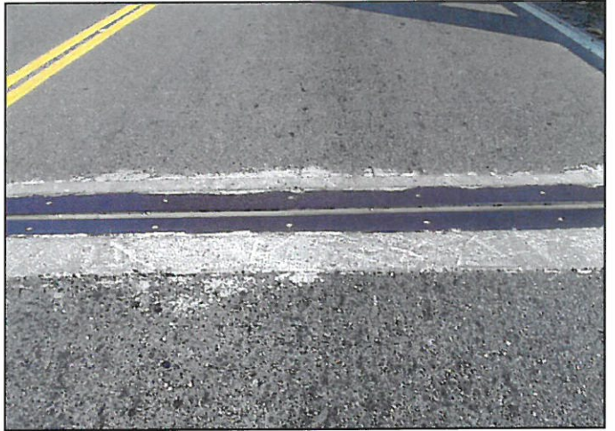
Detail View of Repaired Expansion Joints
