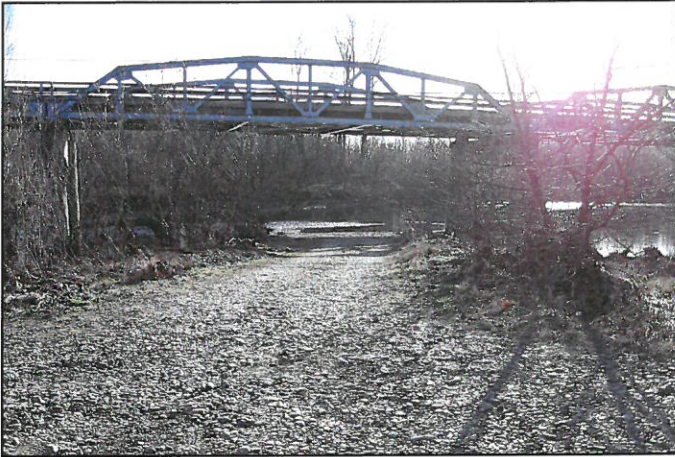
View of Access Road below Bridge, Facing South
