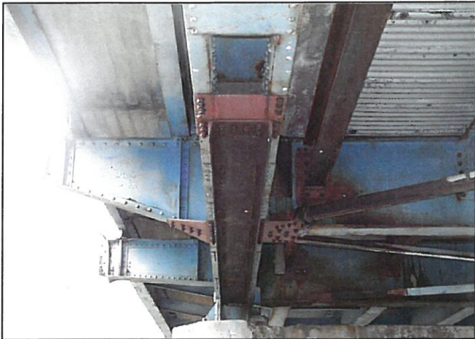
Detail View of Supplemental Replacement Bracing
