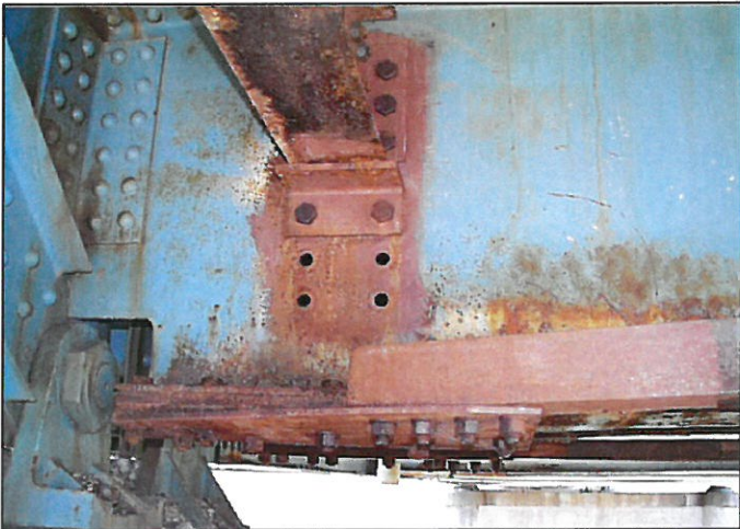
Detail View of Repaired/Replaced Beam Connections
