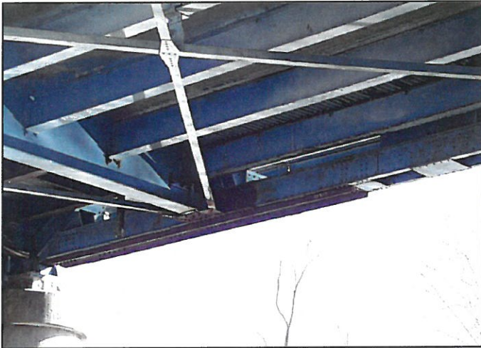
Detail View of Cross Bracing
