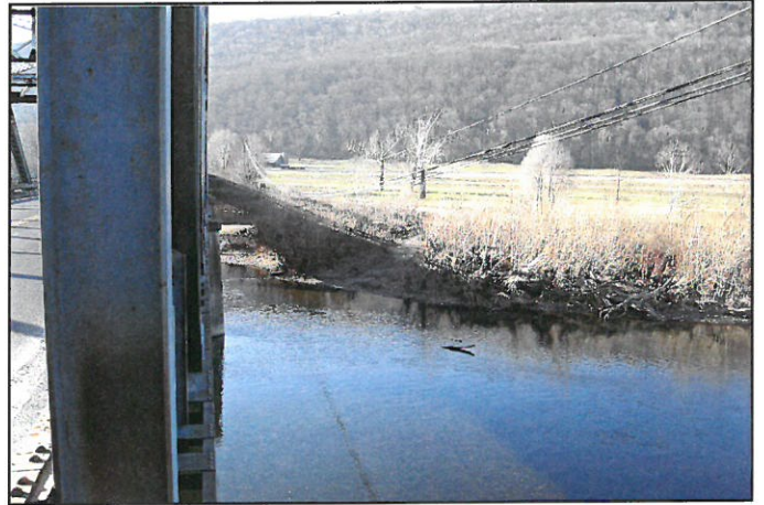
View of Area West of Bridge, Facing West
