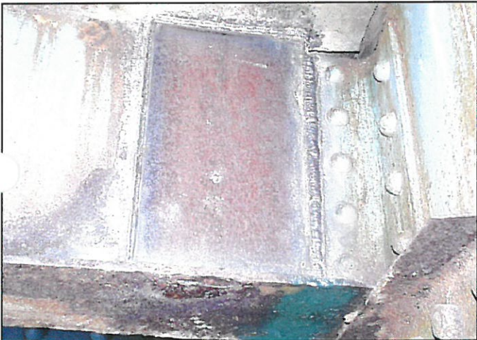
Detail View of Welded Reinforcement Plates
