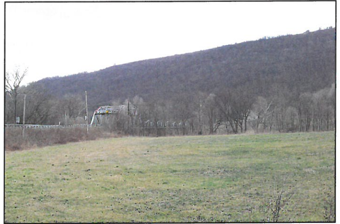
Overview-Romney Bridge Setting, Facing West-Southwest
