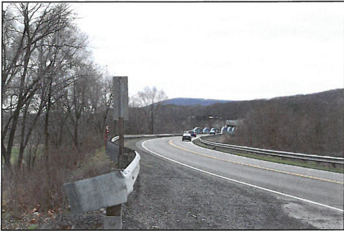
Approach to Romney Bridge from West, Facing East
