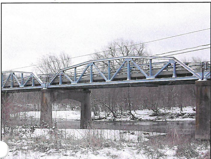
Detail View of Pony Truss, Facing Southeast
