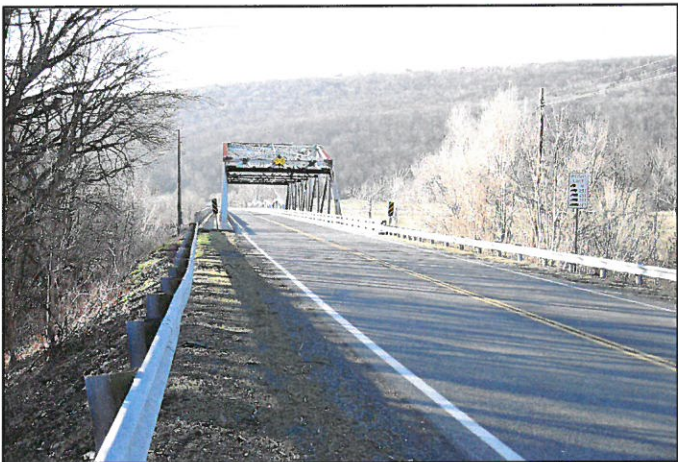
View of Immediate Eastern Bridge Approach, Facing West
