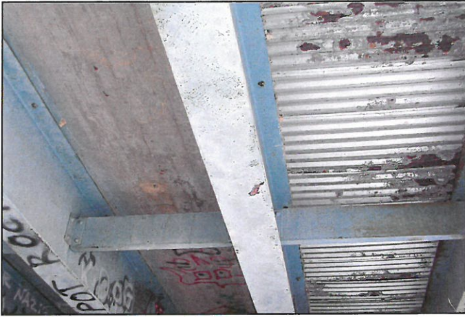
Detail View Showing Repaired Sections under Bridge
