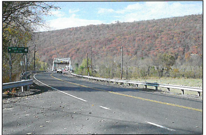
Approach to Romney Bridge from East, Facing West
