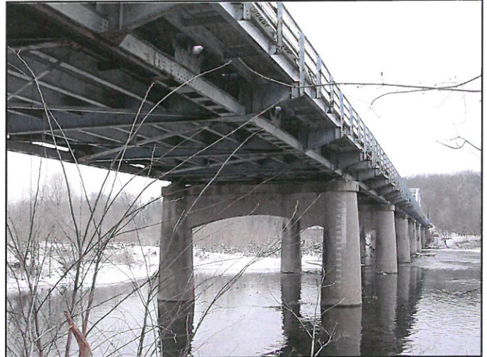
View of Piers and Bridge Underside, Facing East
