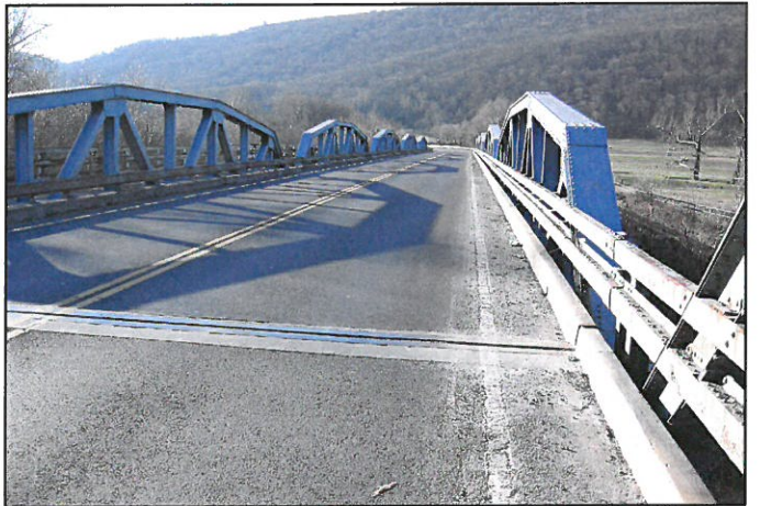
View of Pony Trusses, Facing West
