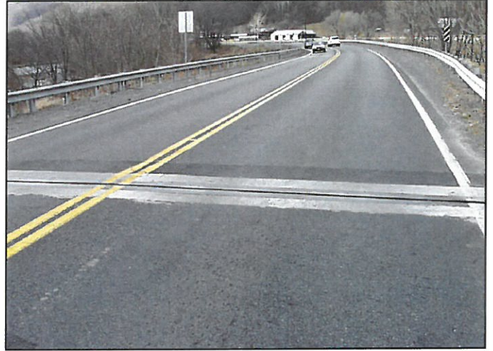
Overview of Expansion Joint Repairs
