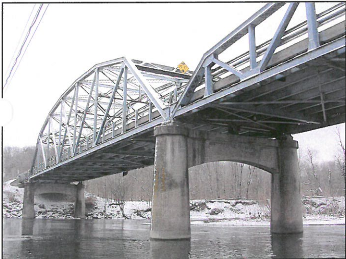
View of Main Span and Underside, Facing East-Southeast
