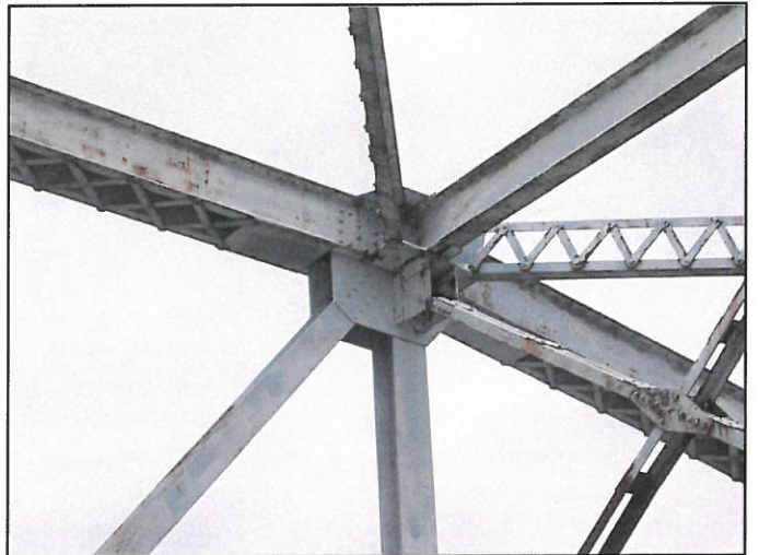
Detail View of Chord/Bracing Connections, Facing East
