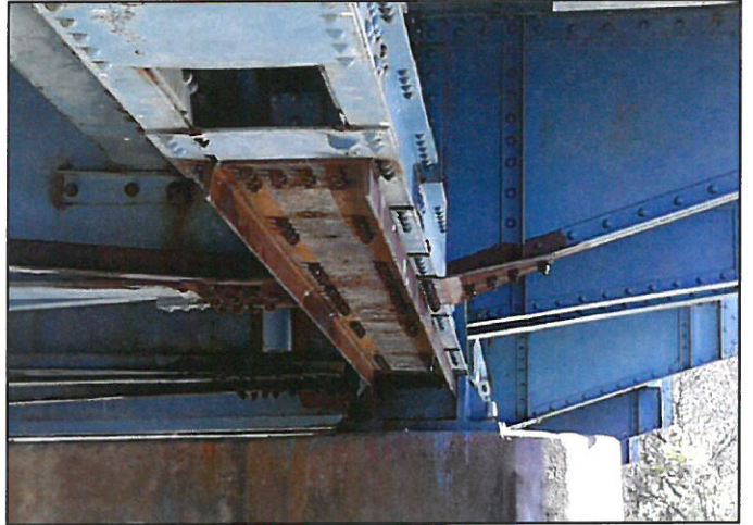
Detail View of Supplemental Replacement Bracing
