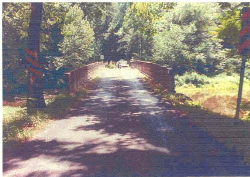
END VIEW OF STRUCTURE LOOKING EAST (Forward)
