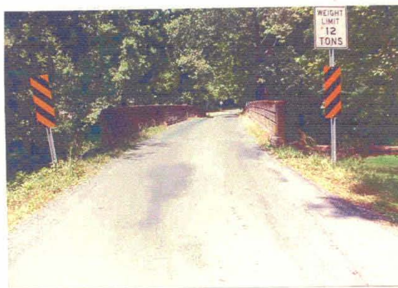
END VIEW OF STRUCTURE LOOKING WEST (Backward)
