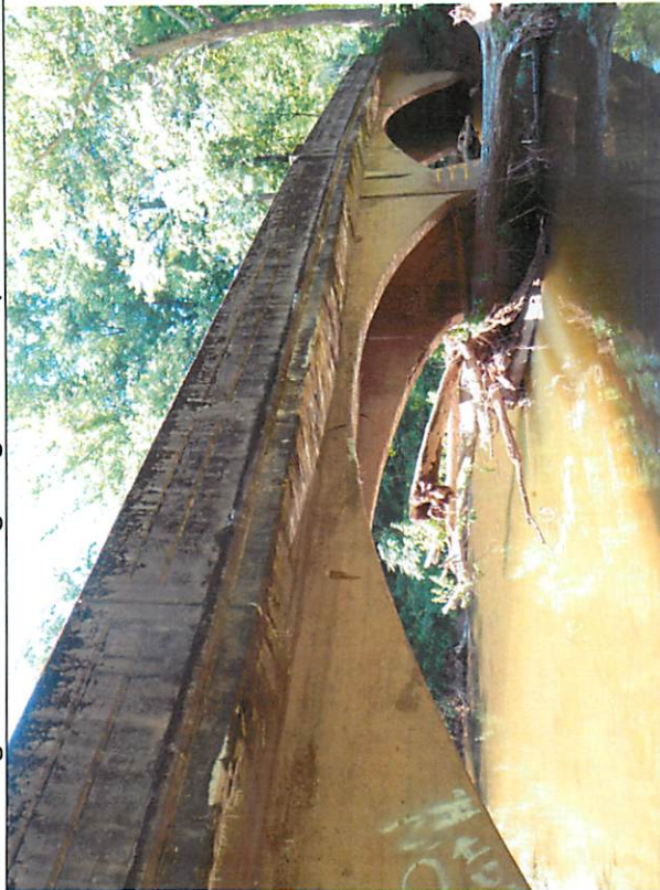
2. Large dead trees lodged against the upstream end of the pier
