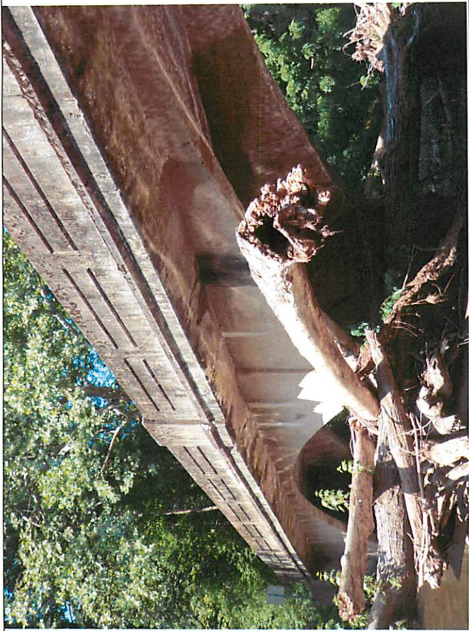
2. Large dead trees lodged against the upstream end of the pier
