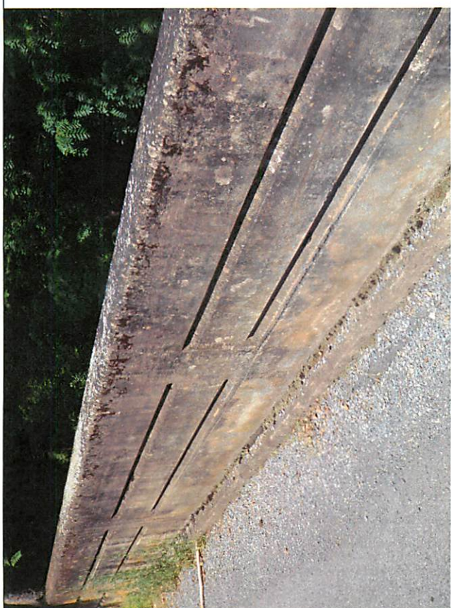
10. Incised parapet wall
