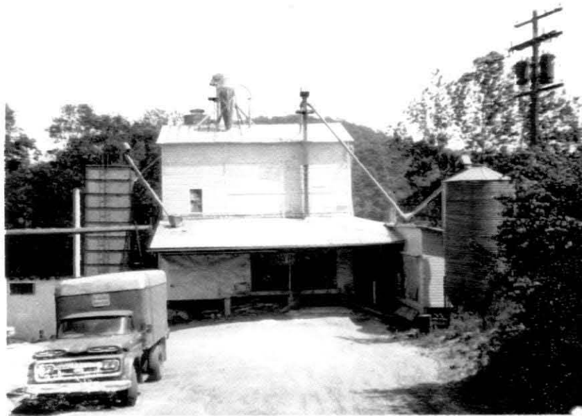
Yellow Spring Mill with the addition of an elevator and a silo.
