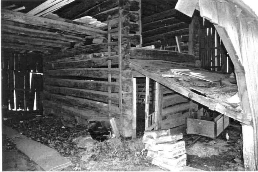
Interior of log barn at site HM-0417
