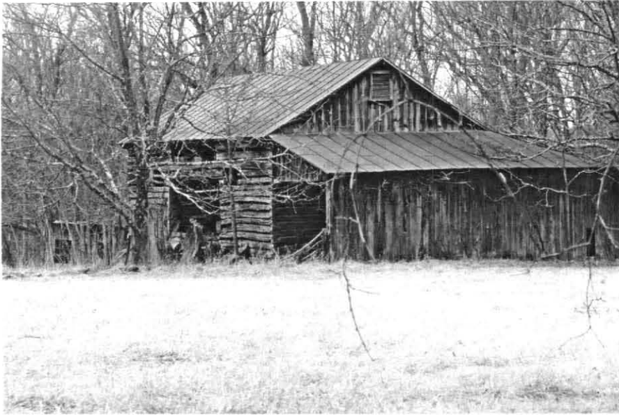
Log barn on Etheridge Etheridge Road.
