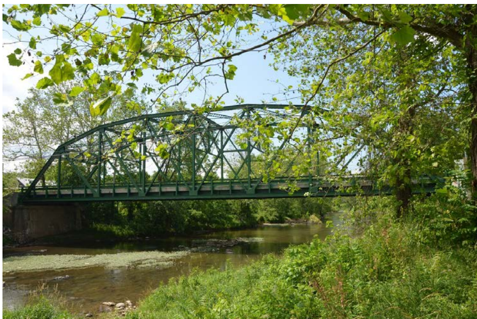
View of the Capon Bridge looking south
