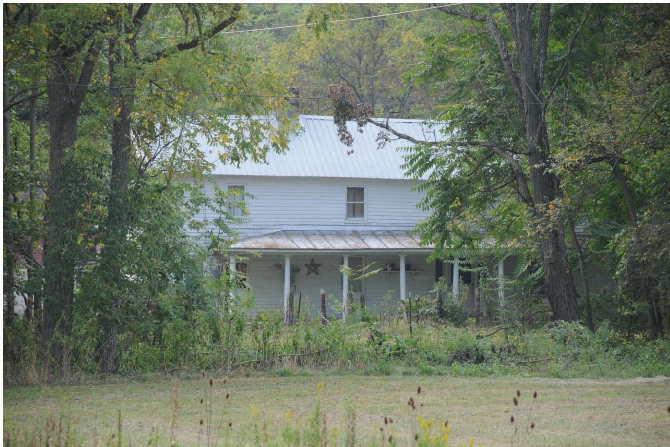
Front of the house at Field No. 10, showing two entries, 1/1 double hung sash and six finely turned Ionic columns.
