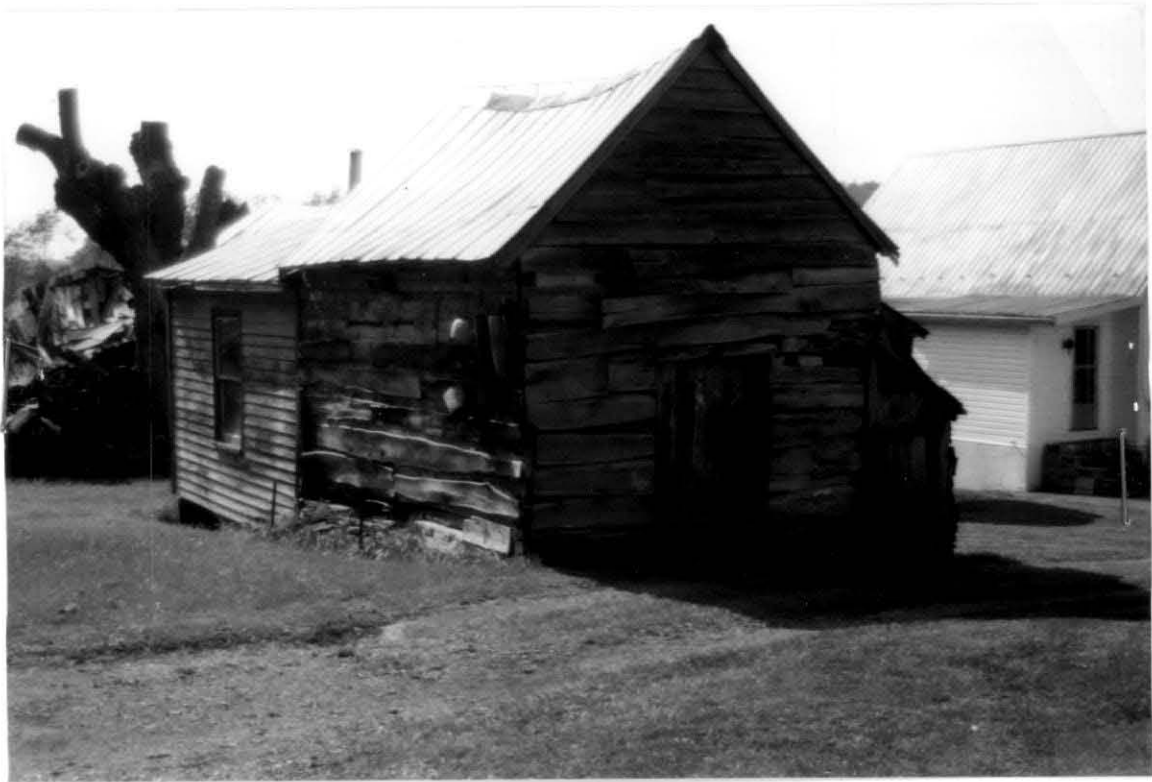
Photo # 9 Woodshop/ workshed Outbuilding #2-3
