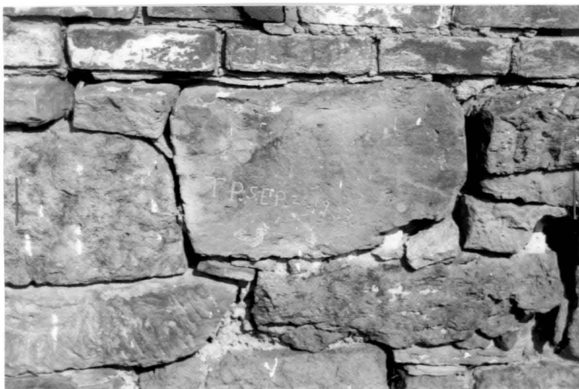
Photo #6 Date of construction in foundation: "T.P. Sep. 26 1903".
