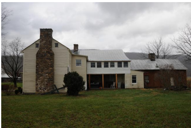
Camera looking west
