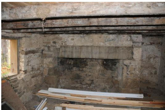
Interior of Kitchen building
