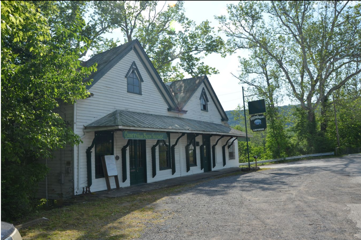
View of the façade of the Store and Post Office looking west
