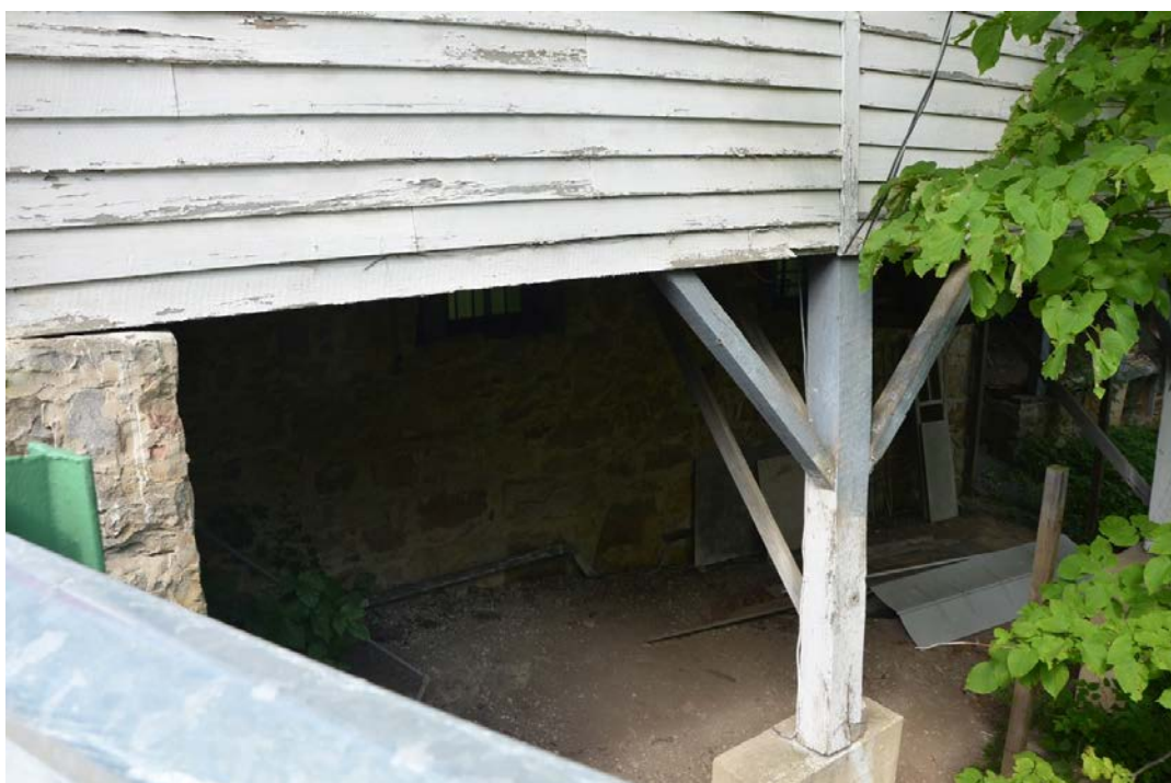
View of the foundations of the Store and Post Office
