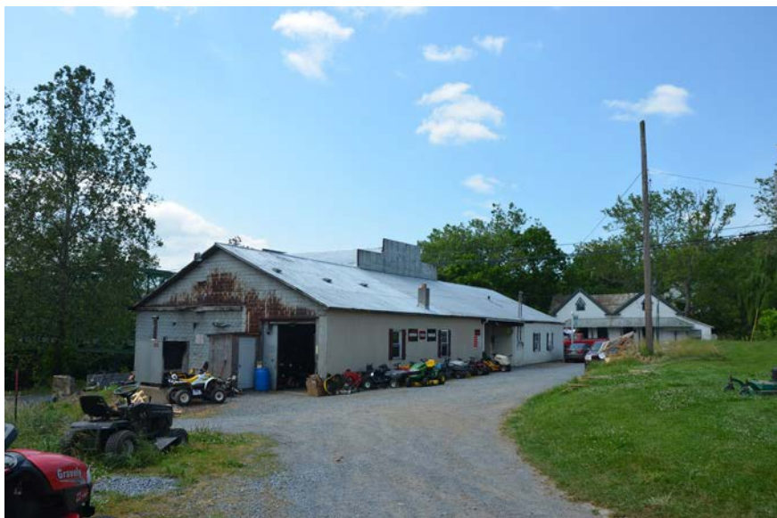
View of the commercial building looking south
