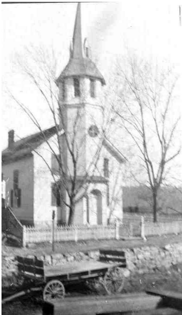
View of the Capon Bridge United Methodist Church ca. 1900
