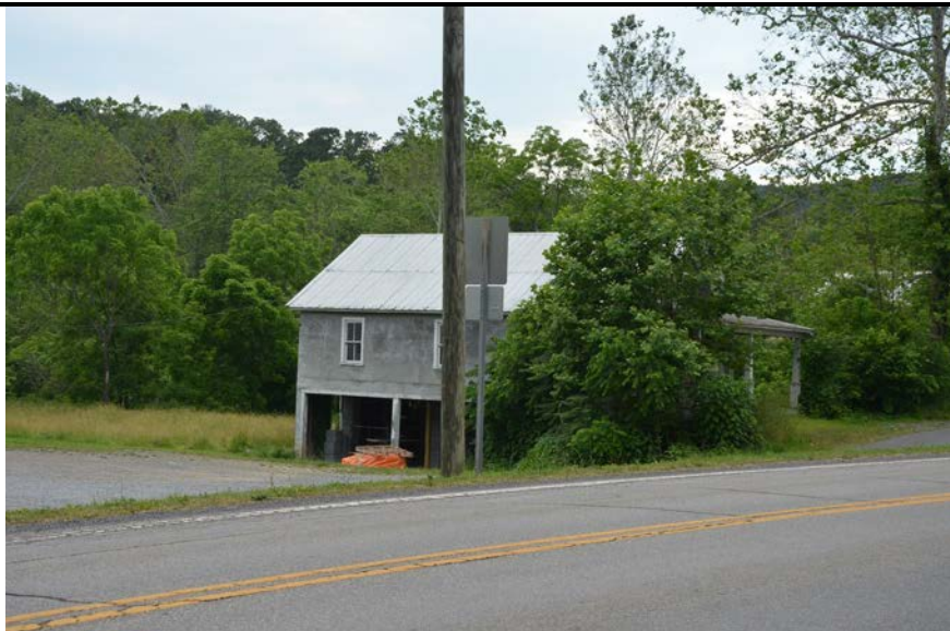
View of east elevation of the Commercial Building looking southwest
