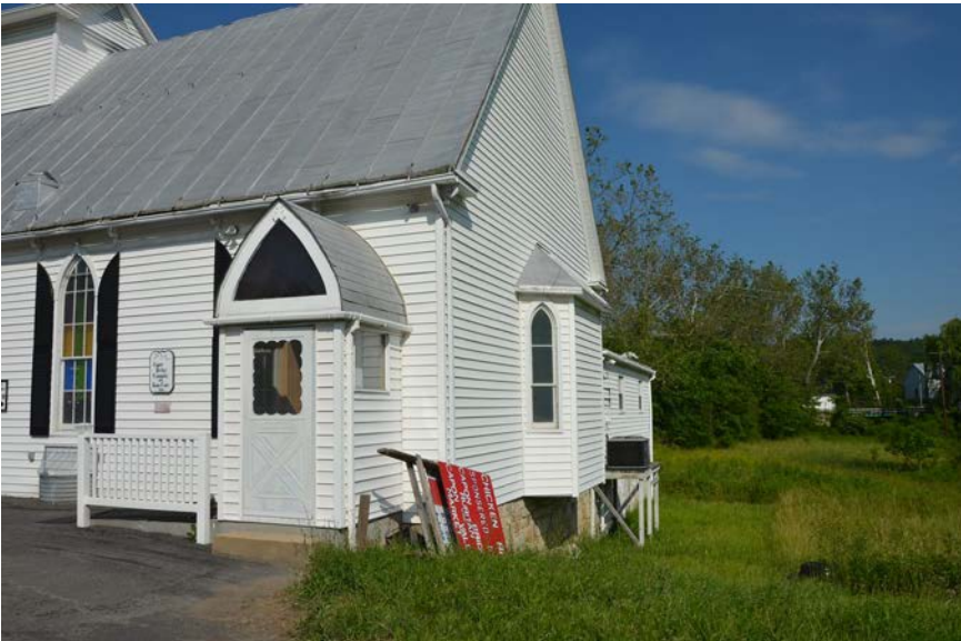
View of the south elevation and coursed ashlar foundation of the former Capon Bridge Presbyterian Church
