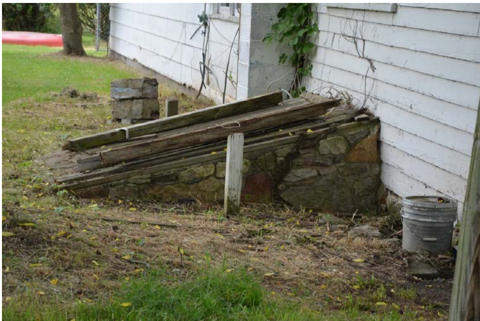
View of the entrance to the partial root cellar on the west elevation looking north
