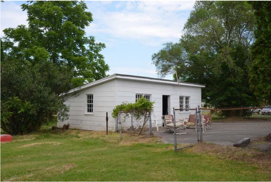
View of the outbuilding located to the north of the rear ell of Frye's Tavern
