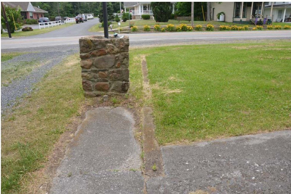
View of the sidewalks and fence base looking south toward U. S. Route 50
