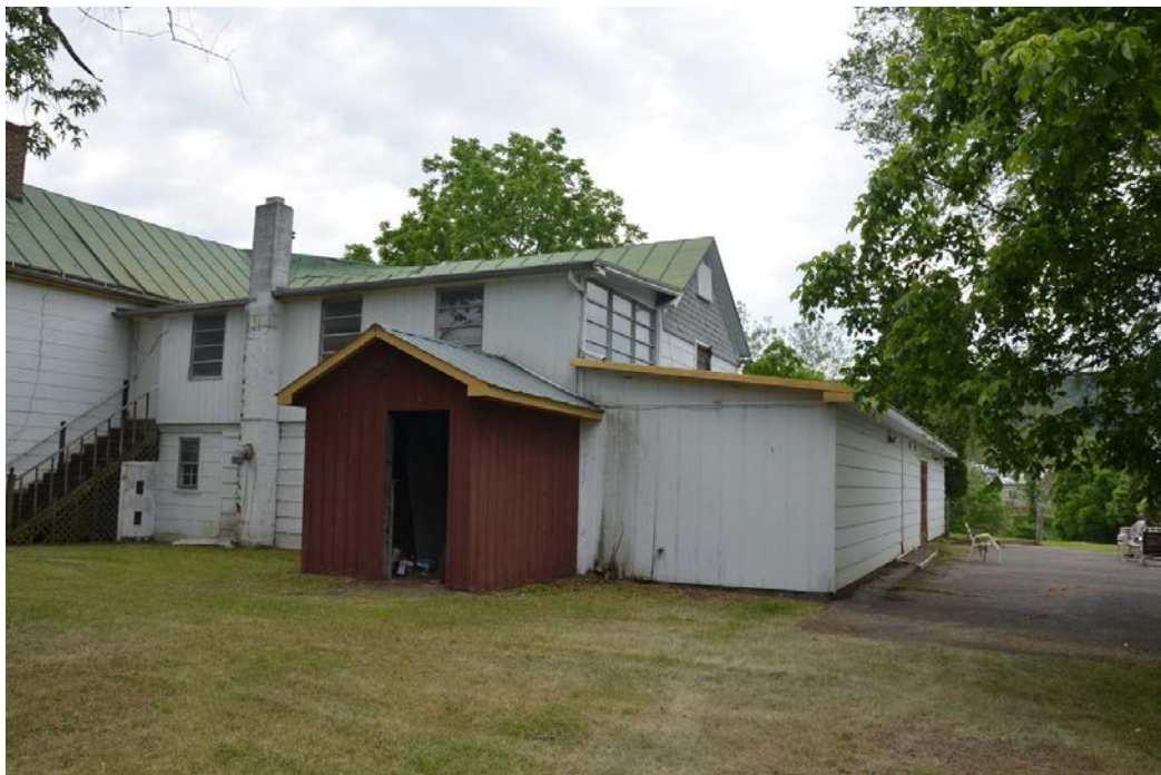
View of the rear ell looking west
