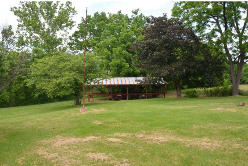
View of the machine shed located to the northwest of Frye's Tavern
