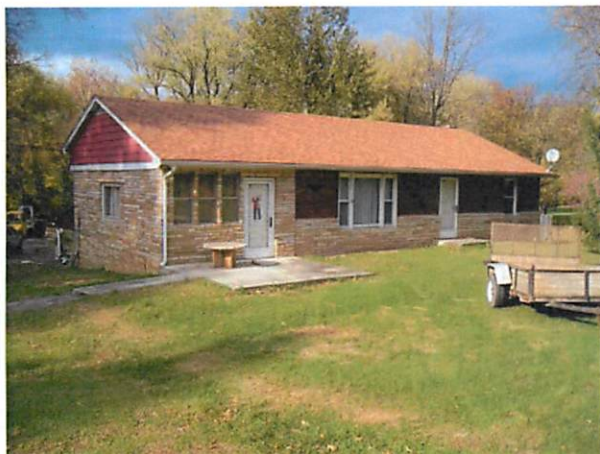
Photo 1: Front (southeast) elevation.
