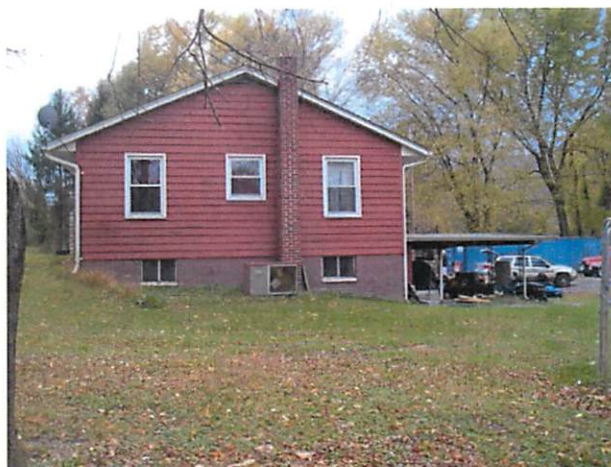
Photo 4: Right side (northeast) elevation.
