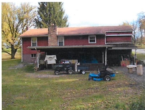
Photo 3: Rear (northwest) elevation.
