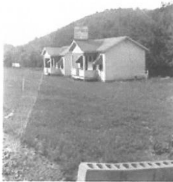
Cabins being built
