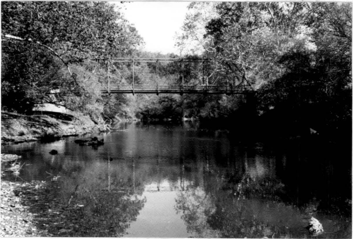
Plate 3. Two Lick Creek Bridge. View to north (downstream).
