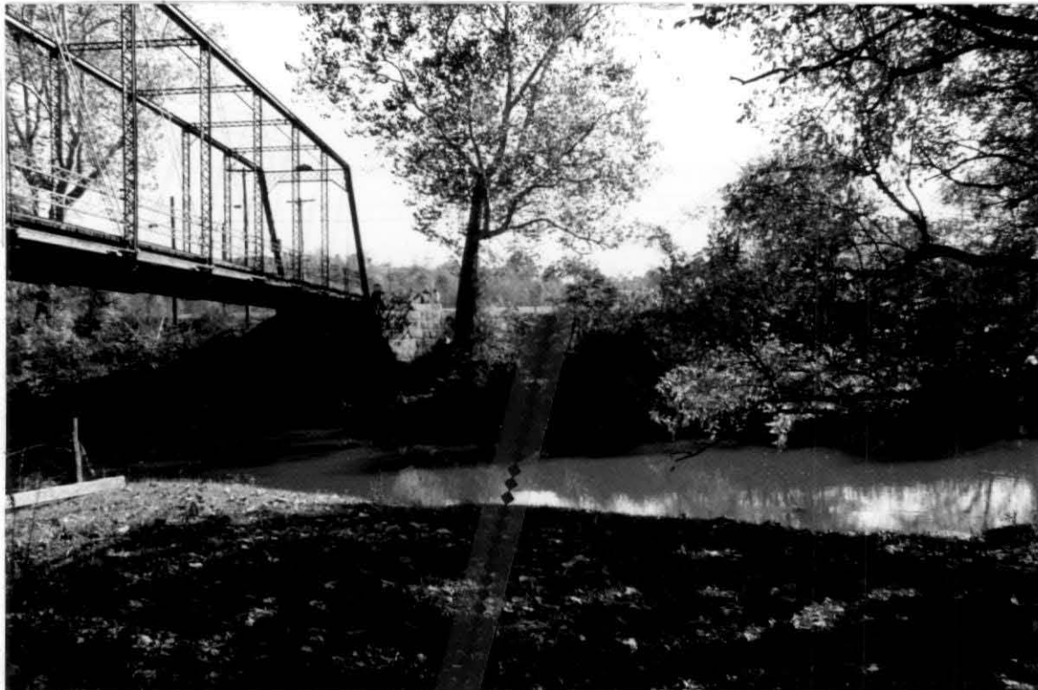
Plate 6. Approximate center line of new bridge. View to east.
