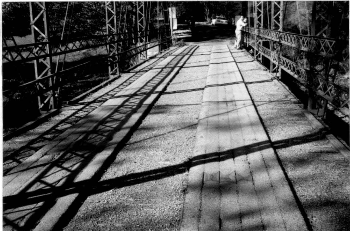
Plate 2. Bridge deck. View to west.
