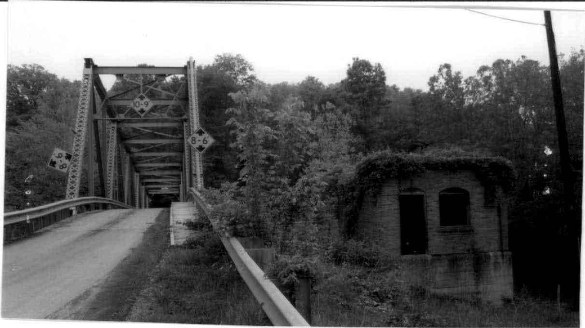
Photo of truss bridge and pump house. Facing Northwest.
