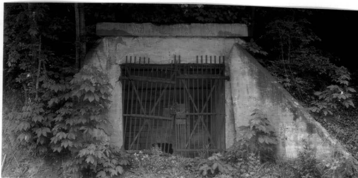
Photo of Entrance Adit. Facing Northwest.
