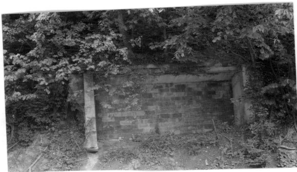
Photo of Exit Adit. Facing Northwest.
