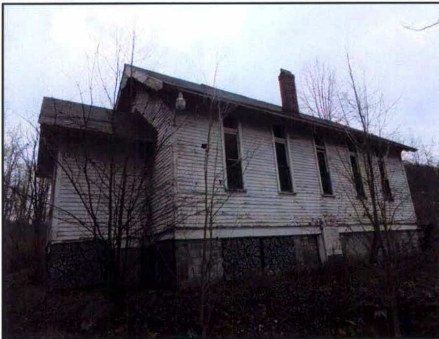
View of the northwestern elevation, facing south.
