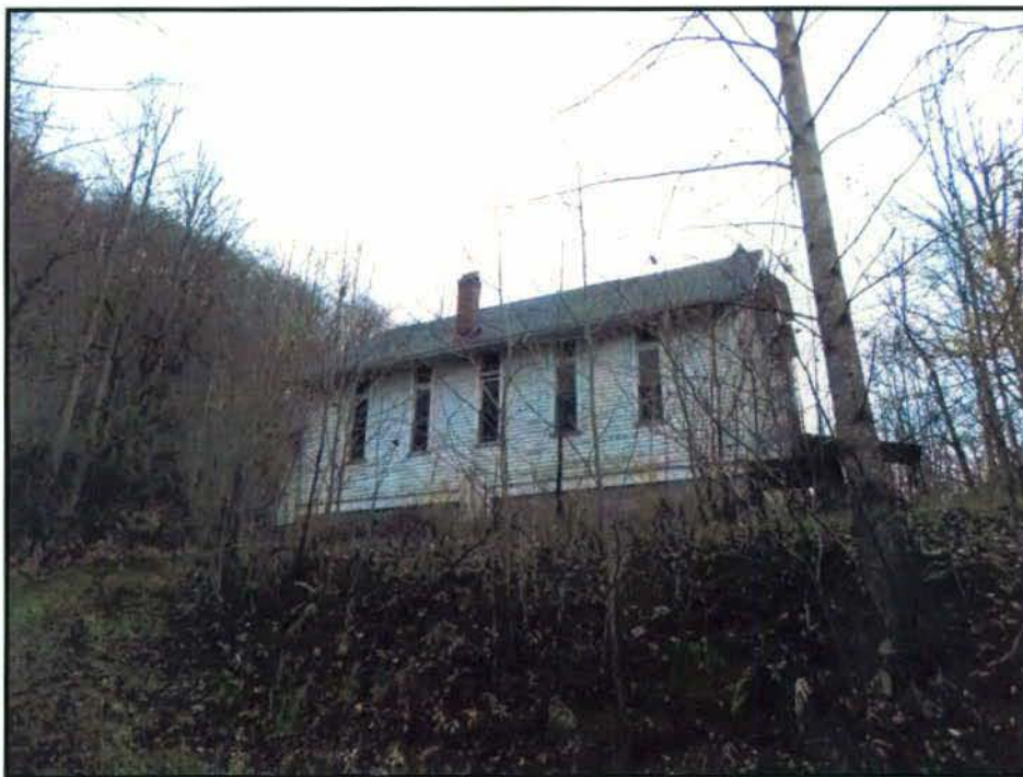
View showing the northwestern elevation and setting, facing southeast.
