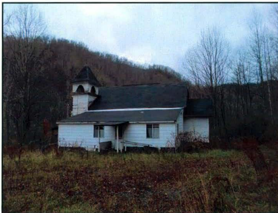
View of the southeastern elevation, facing northeast.
