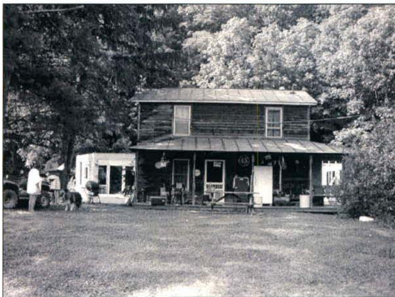
Photograph of the façade of the Judy Harman House, facing north.
