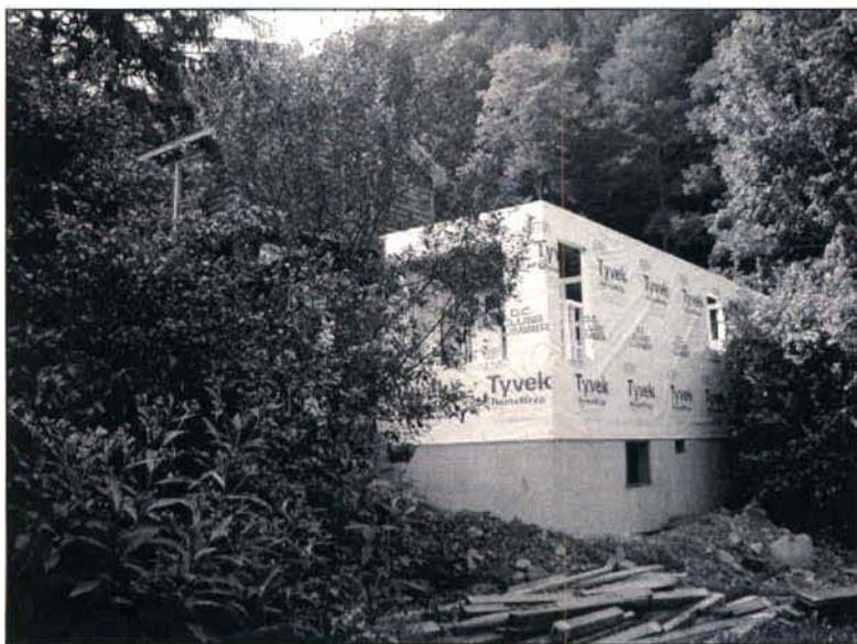
Photograph of ongoing renovations at the Judy Harman House, facing northwest.
