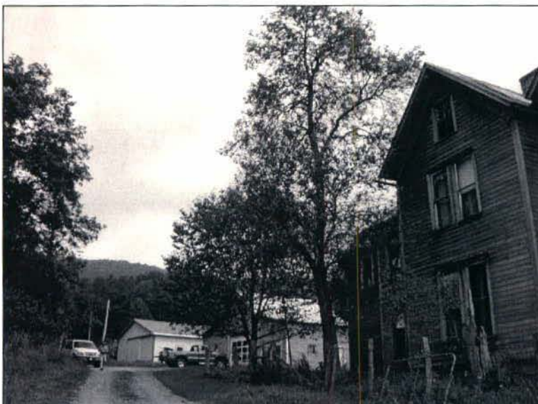
Photograph of the Snyder House showing Features J (modern) and I behind it, facing north.
