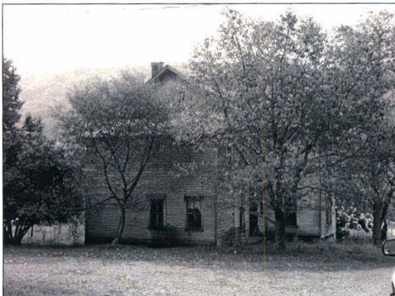
Photograph of the rear elevation of the Snyder House, facing south by southeast.
