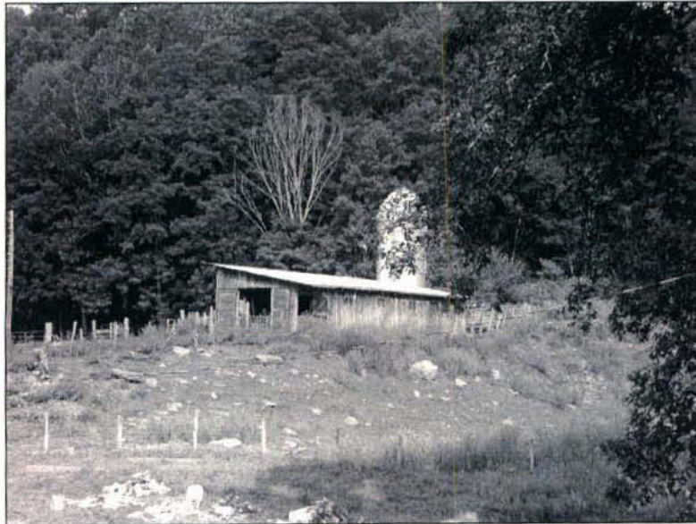
Photograph of shed roof barn and associated silo (Figure G) near Snyder House, facing northwest.
