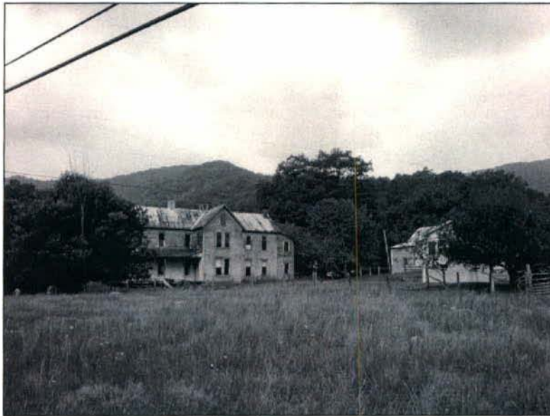
Photograph of the east side elevation of the Snyder House showing modern home and Feature I in foreground, facing east by northeast.
