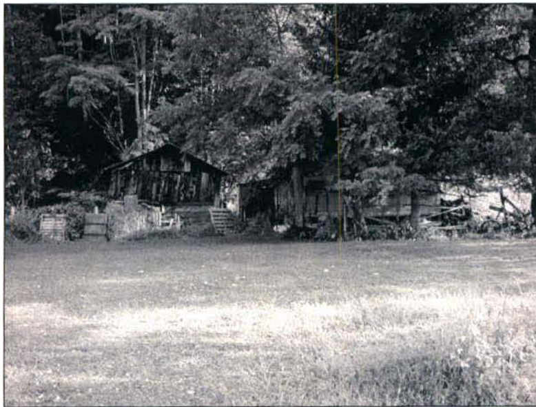
Photograph of dependencies (Feature D) found in association with the Anna Harman House, facing north.
