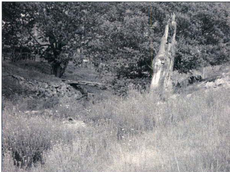
Photograph of small footbridge (Feature Q) located between Snyder House and 19 th century barn, facing north.
