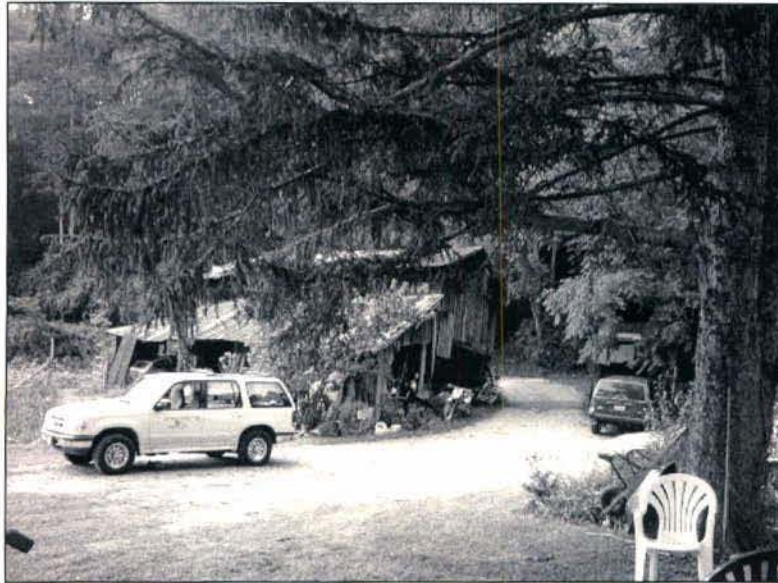
Photograph of the gable-roof dependency (Feature N) associated with the Judy Harman House, facing northwest.
