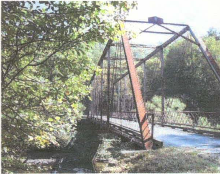
Photo #1 Elevation View Looking upstream and right
