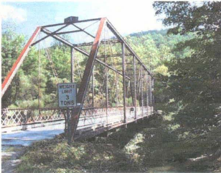
Photo #2 Elevation View Looking downstream and left
