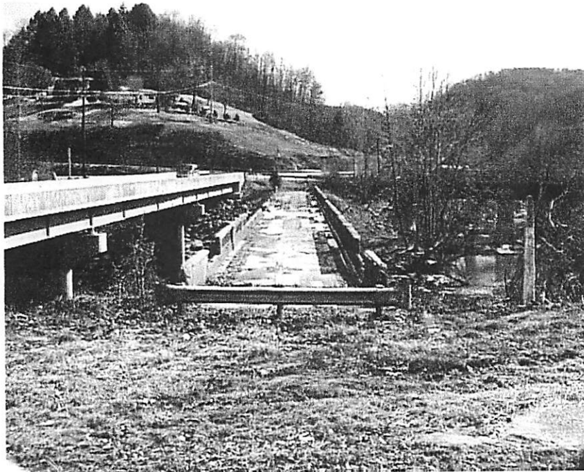
A VIEW OF THE GUARDRAIL BARRICADE FROM ABUTMENT ONE.
