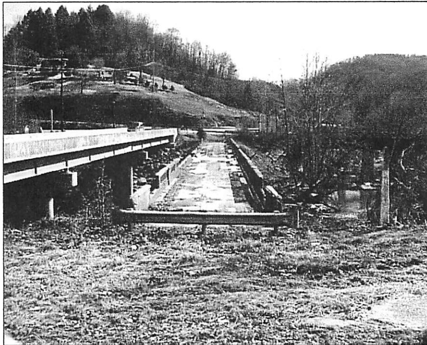
END VIEW LOOKING FROM ABUTMENT ONE
