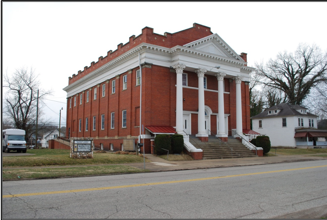
Figure 43. East and façade (north) elevations of the Sixteenth Street Baptist Church, looking to the southwest.
