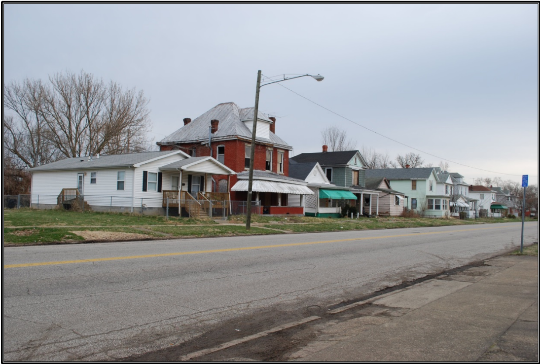
Figure 45. Residences along the north side of Ninth Avenue near the Sixteenth Street Baptist Church, looking to the northeast.
