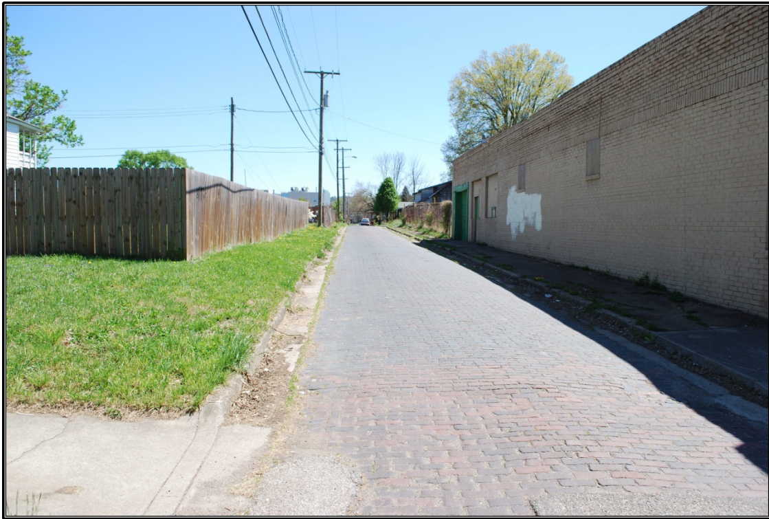
Figure 39. Brick pavers along Fourteenth Street looking to the south from Tenth Avenue.
