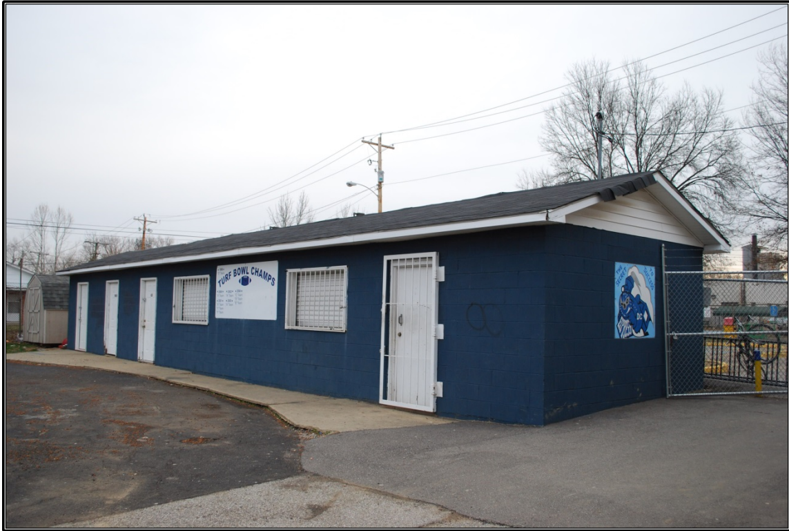
Figure 61. Restroom and concession stand building adjacent to the athletic field, looking to the northeast.
