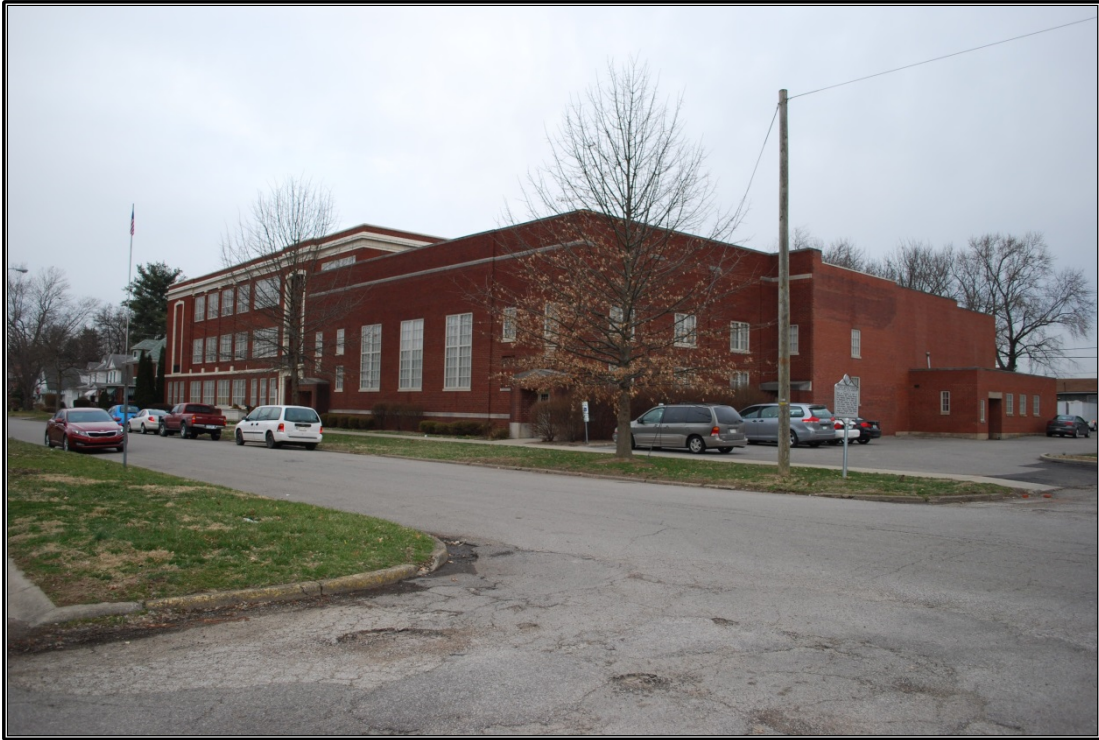
Figure 56. Façade (south) and east elevations of the Douglass Junior and Senior High School, looking to the northwest.
