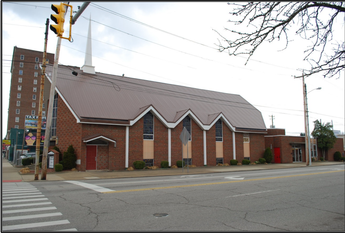
Figure 28. Façade (north) and west elevations of First Baptist Church, looking to the southeast.
