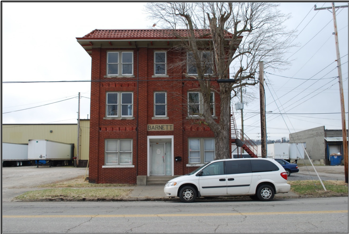
Figure 24. Façade (north) elevation of the Barnett Hospital and Nursing School, looking to the south.
