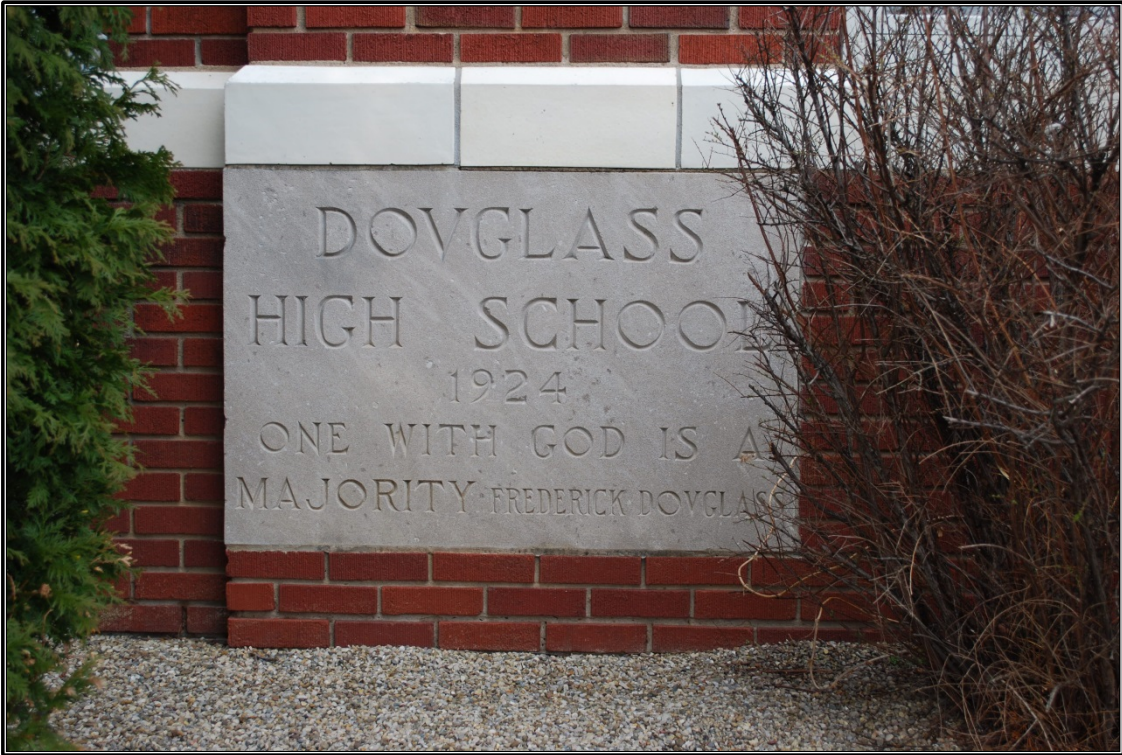
Figure 55. Detail of the cornerstone at the southwest corner of the main block.
