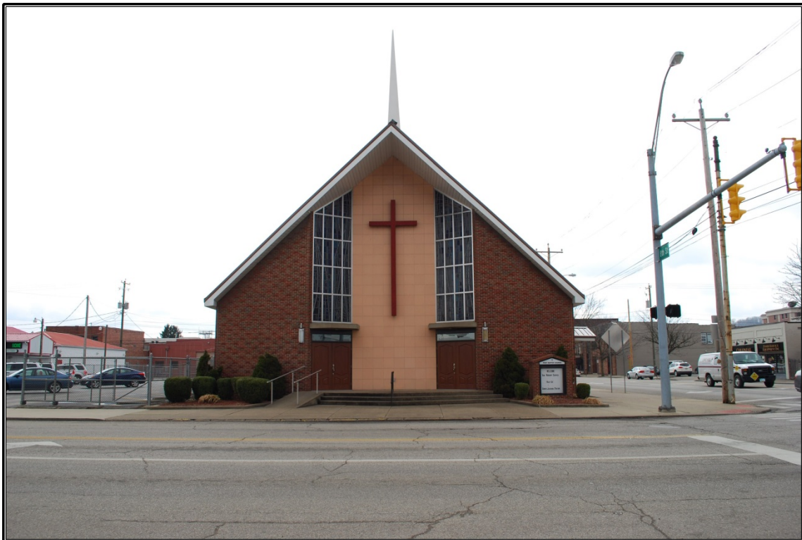
Figure 27. Façade (north) elevation of First Baptist Church, looking to the south.
