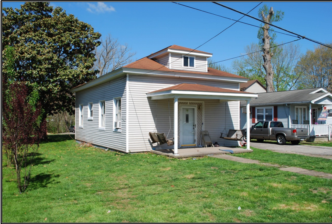
Figure 15. South and façade (east) elevations of the former Barbourville Colored School, looking to the northeast.
