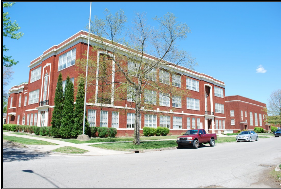
Figure 52. West and façade (south) elevations of the Douglass Junior and Senior High School, looking to the northeast.
