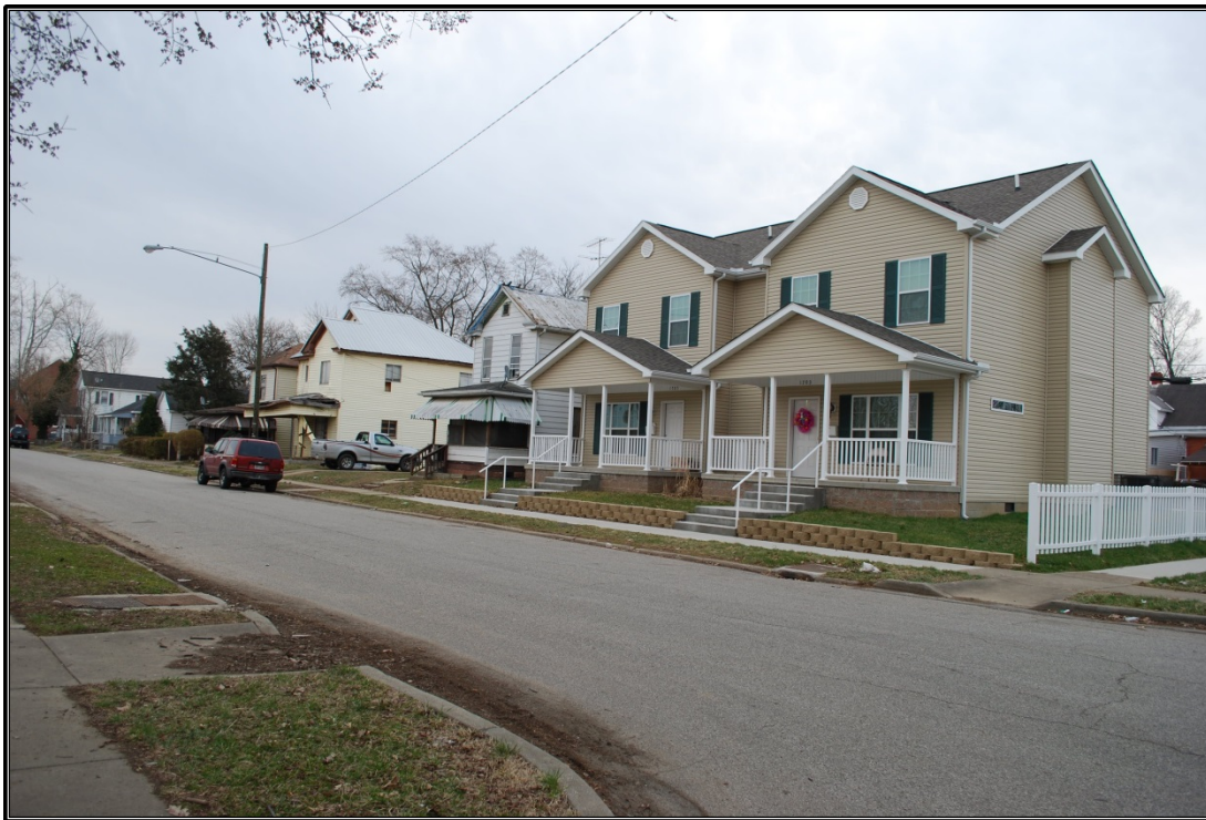
Figure 36. Recent house construction and older dwellings along the south side of Artisan Avenue from the intersection with Seventeenth Street, looking to the southeast.
