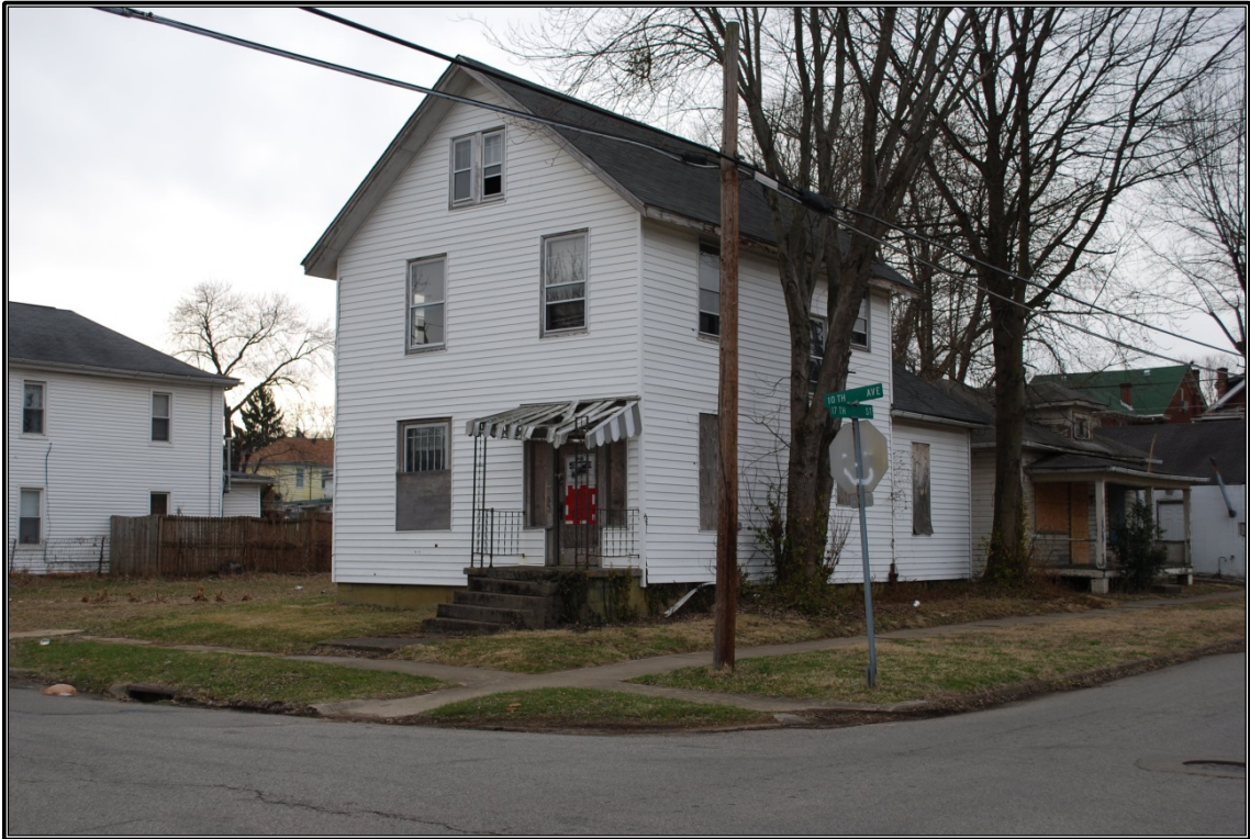
Figure 64. Façade (north) and west elevations of the Memphis Tennessee Garrison residence, looking to the southeast.
