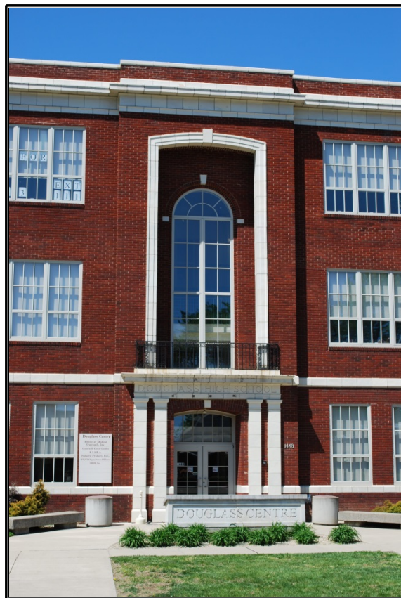
Figure 53. Detail of the façade's (south) elevation entrance to the Douglass Junior and Senior High School, looking to the north.
