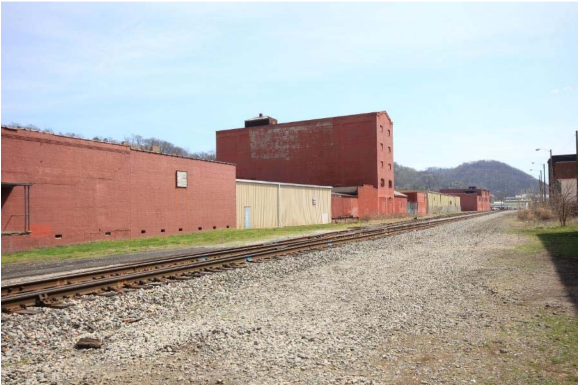
2. Railroad behind resources KA-4649-0073, 72, 71 and 70, taken from Morris Street.
