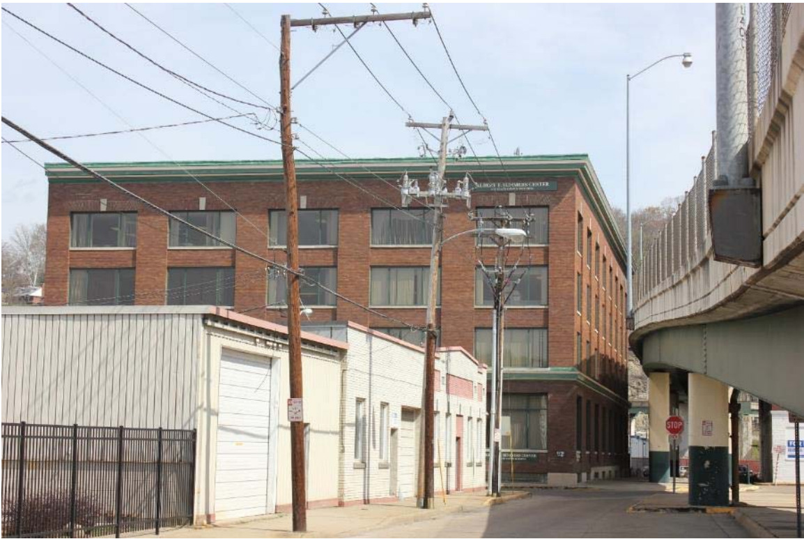
1. Interstate Ramp along Brooks Street at Smith Street; KA-4649-0012 and 0013.
