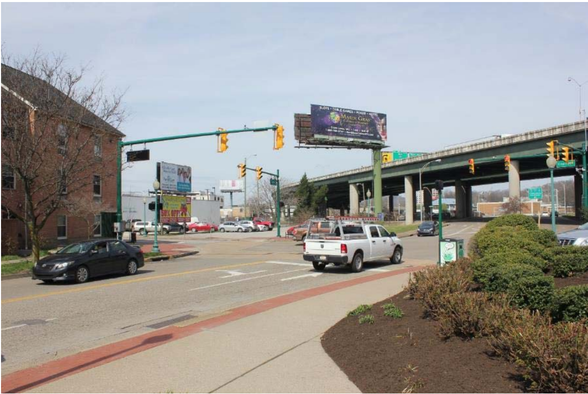
3. Intersection of Capitol and Smith Streets showing interstate, looking west from Capitol Market.
