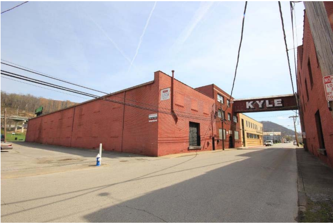
7. Looking southeast on Hansford Street at McJunkin/Kyle Furniture, resources 0053-0055.
