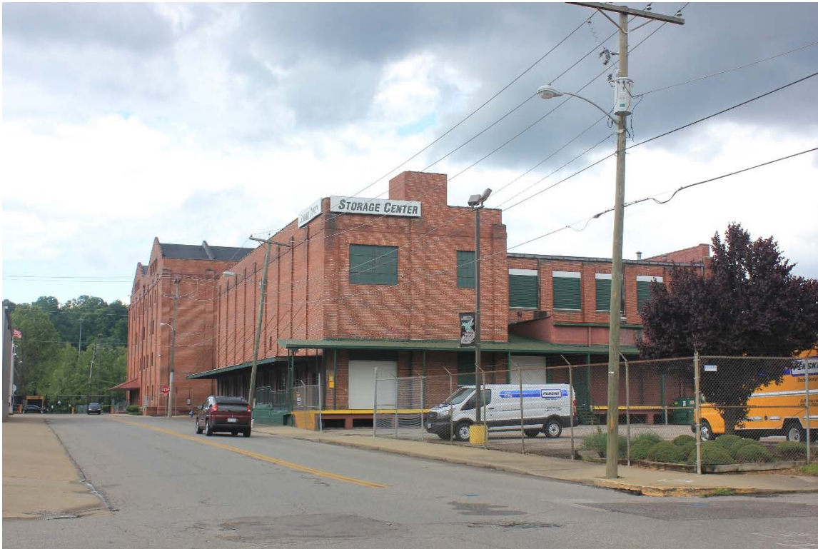
9. Looking north on Piedmont Road at former Diamond Ice & Coal facilities, KA-5488 and 5502.
