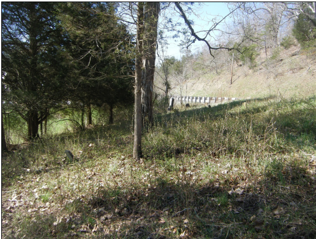
Photograph of 46-HM-140, looking southwest.
