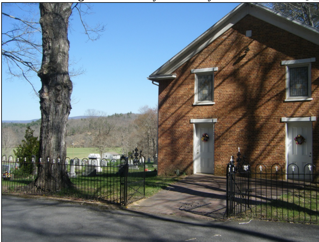
Photograph of 46-HM-190, looking east.
