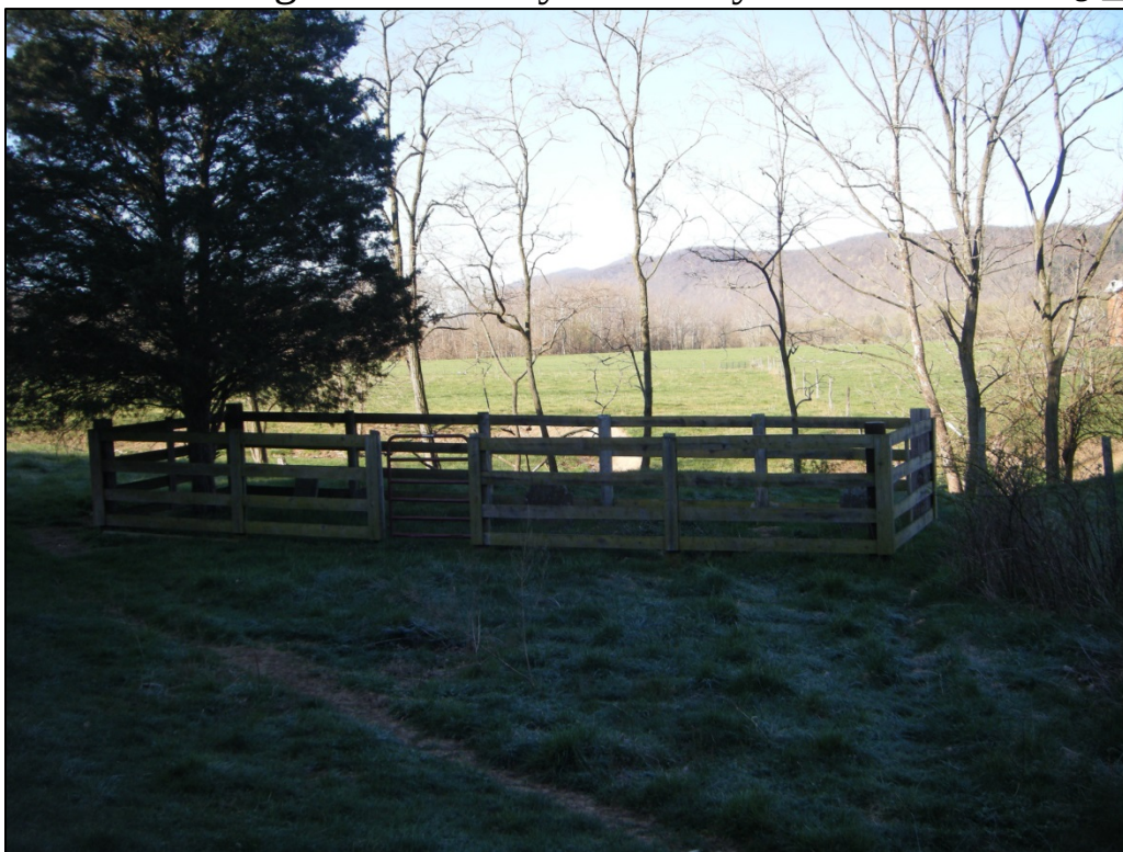
Photograph of 46-HM-200, looking west.
