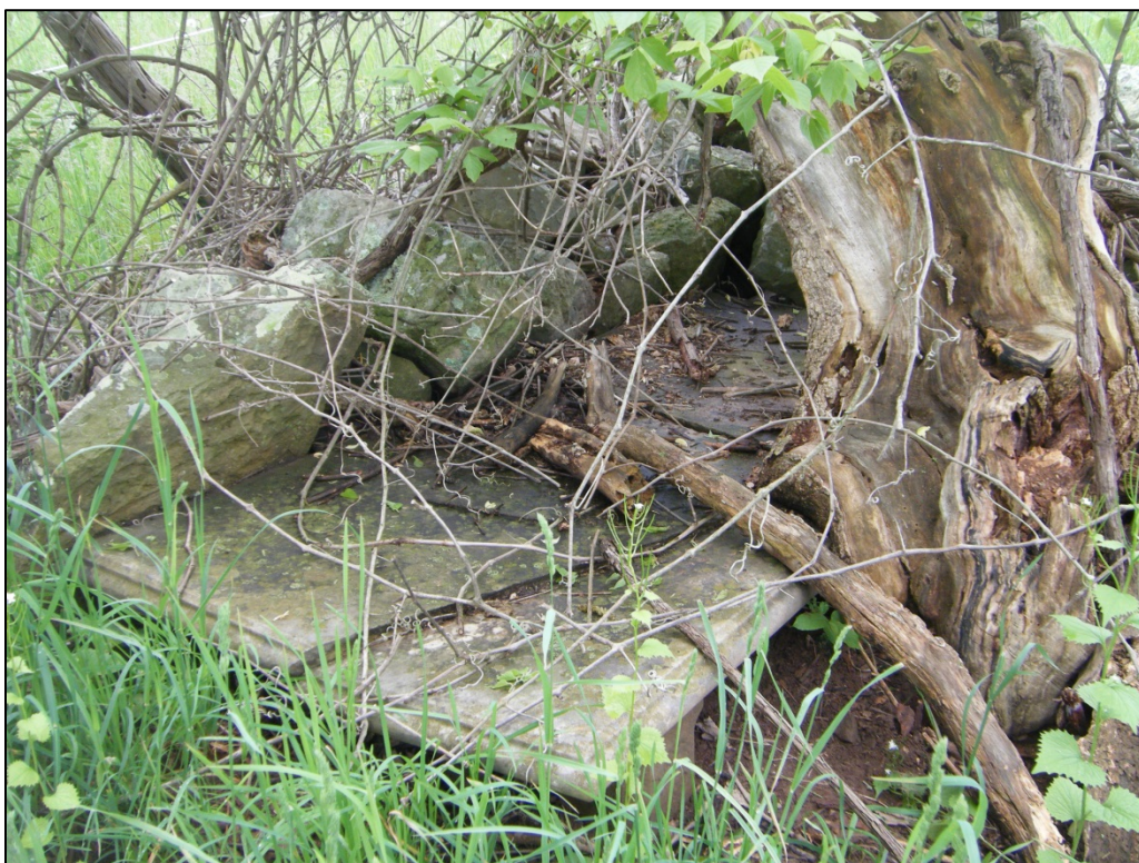
Photograph of a cracked and overgrown crypt documented at 46-HM-240.
