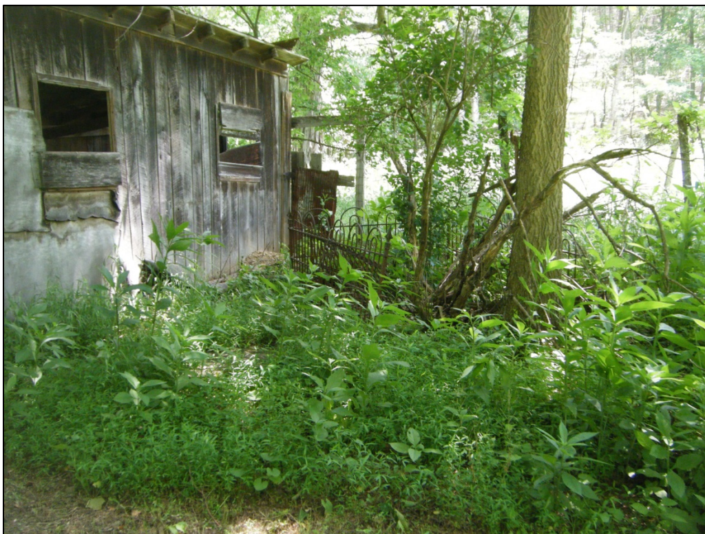
Photograph of 46-HM-248, looking east.
