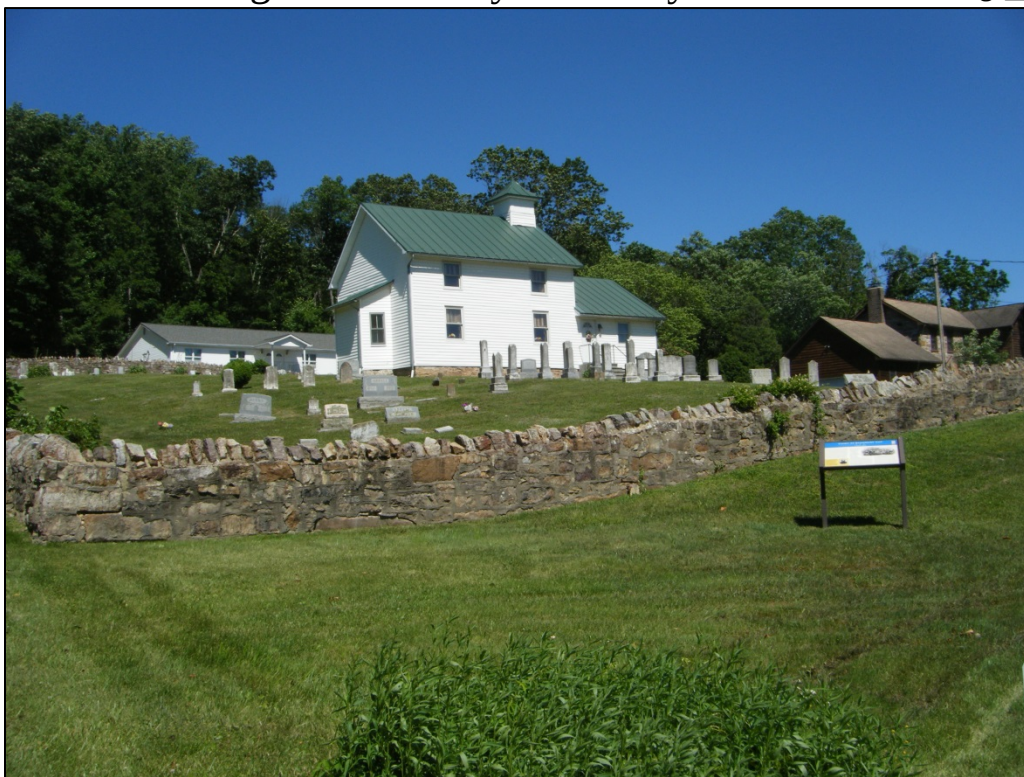
Photograph of 46-HM-251, looking east.
