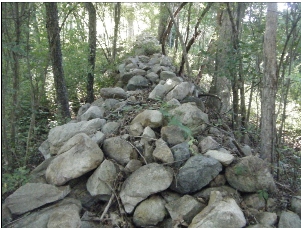
Photograph of the rock wall at 46-HM-252, looking west.
