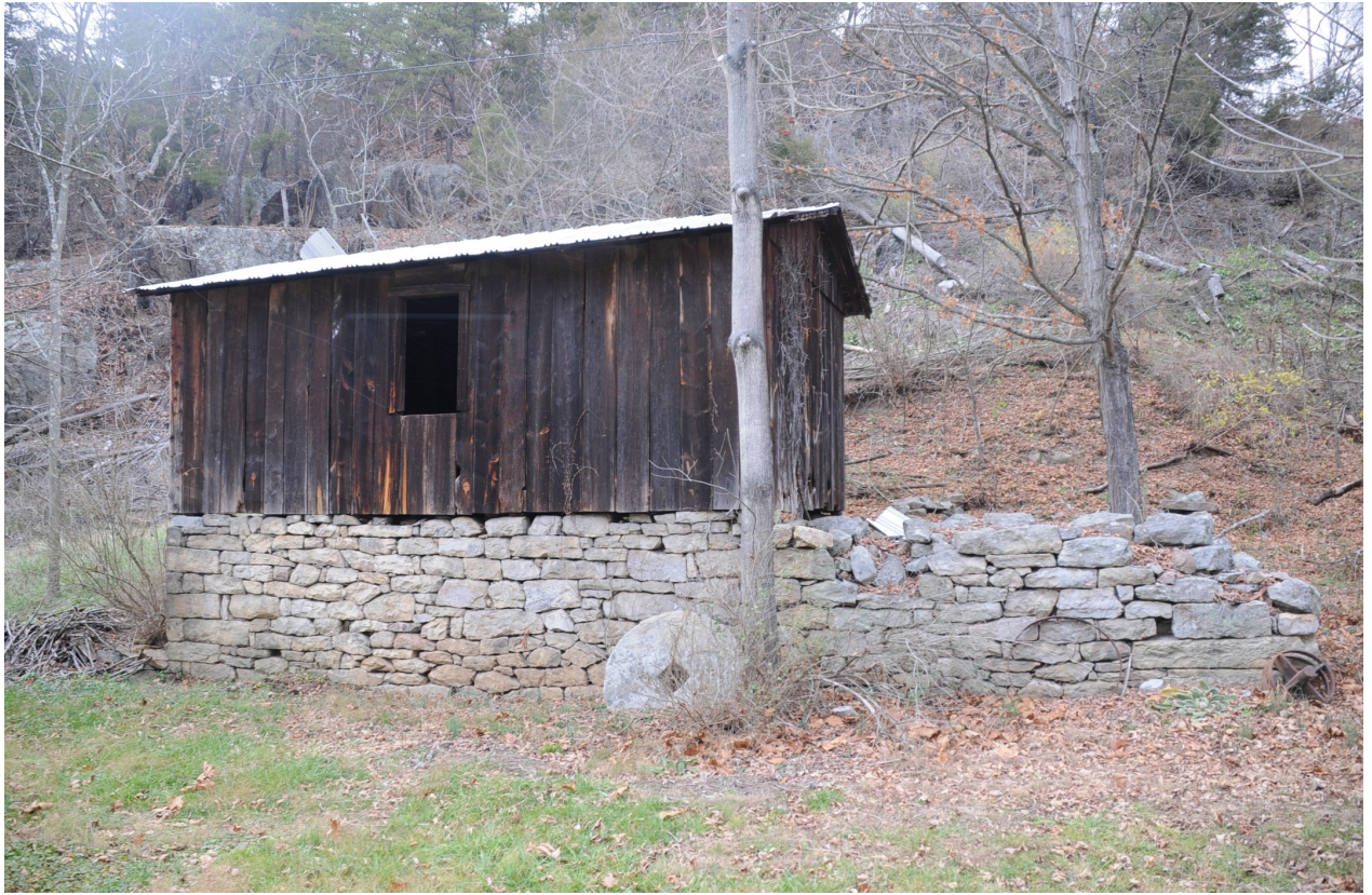
Photo 9: Miller Mill Foundation (#6a)
