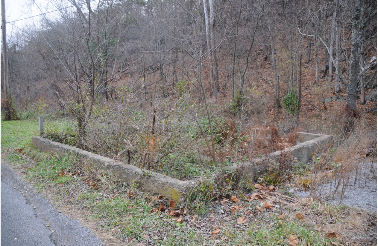
Photo 5: Shanholtz Mill Foundation (#10)
