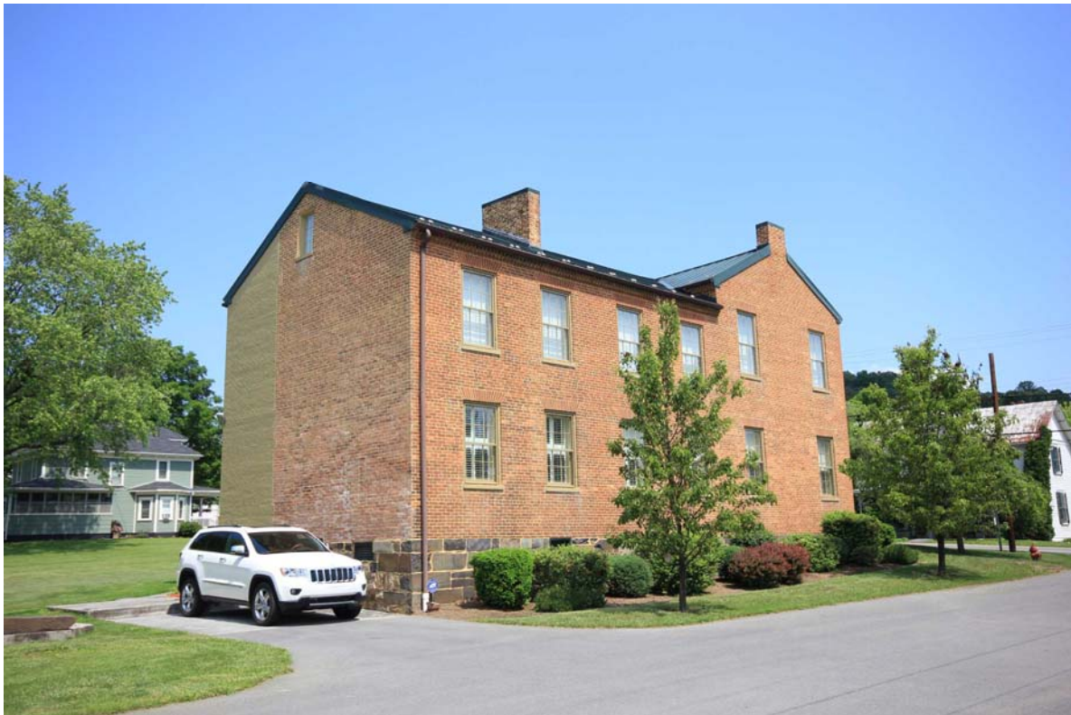
Photo 6: Oblique view of side elevation of house looking north
