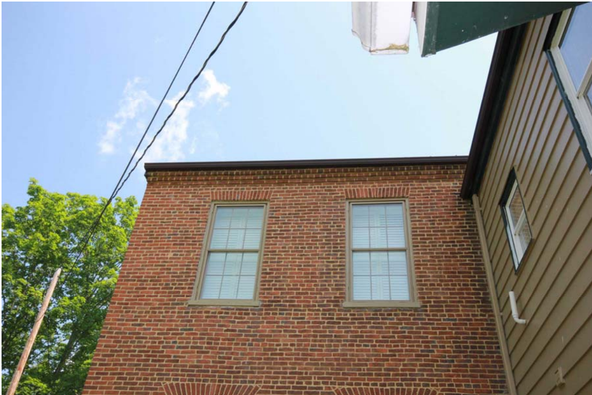
Photo 9: Detail of windows and brick corbelling
