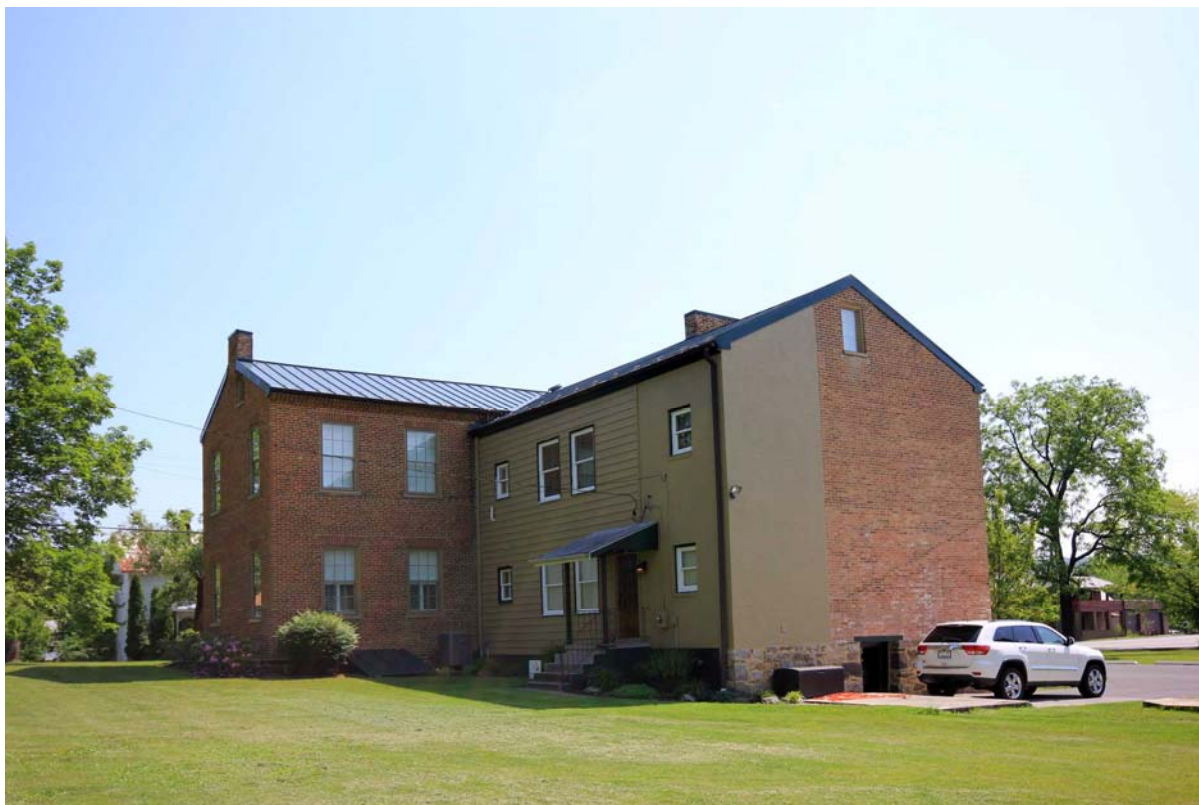
Photo 4: Oblique view of rear of house looking east
