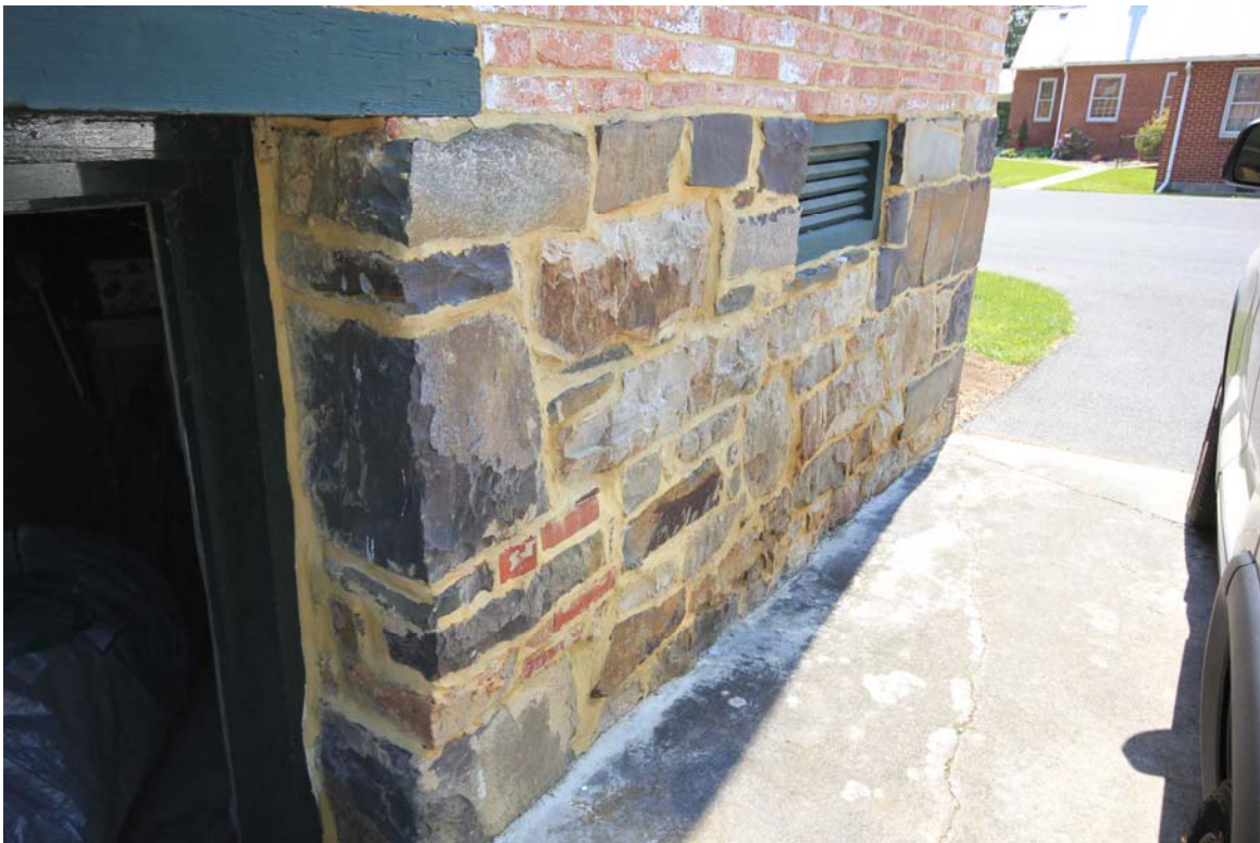
Photo 10: Detail of random coursed sandstone foundation at cellar entrance
